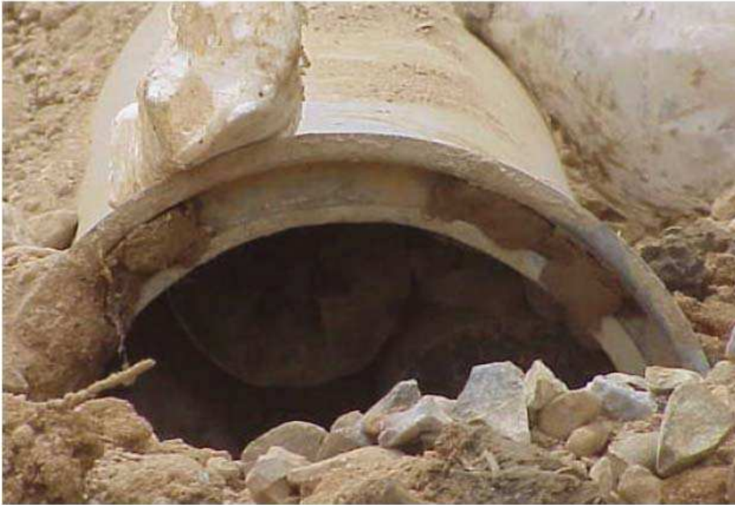
Projectiles inside of a roadside culvert pipe
