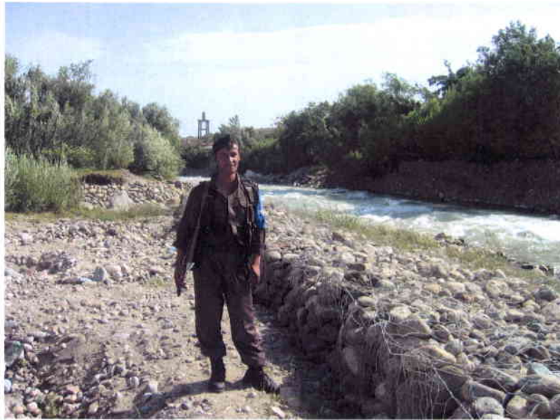
Figure 1: Stones available on the river bed were used to fill the gabions.
