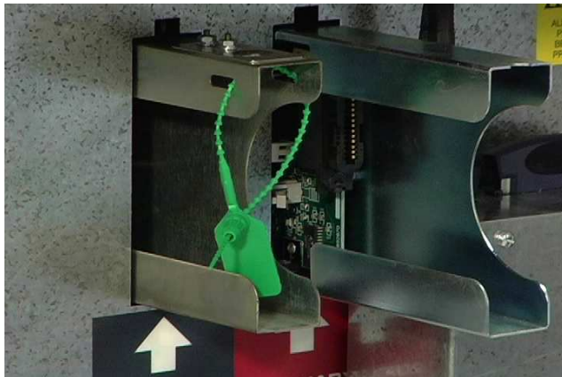
Figure 13: A green plastic-strap seal in the Results Port of an AVC Advantage, exactly as installed there by Union County, New Jersey. This seal is supposed to prevent removing the circuit-board cover without breaking the seal, but in fact it is possible to remove the circuit-board cover without removing the seal.
