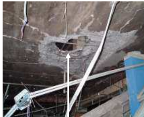
Exit Crater of the seat of explosion
