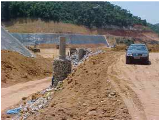
3. Pictures taken in April and September, 2003 – gas drainage system
