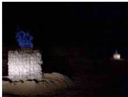
FIGURE 5 Gas wells already burning at Adrianópolis landfill
