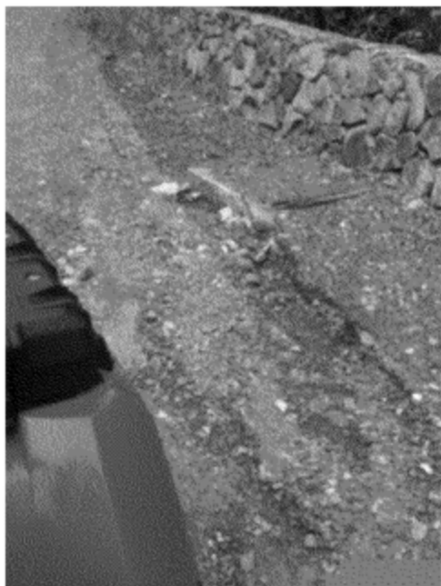
drainage for roads
