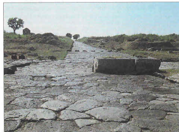
Below: this stretch of Roman road at Vulci, Italy, still survives in remarkably good repair. These essential arteries of communication were solidly constructed to withstand the elements and provide an all-weather surface.
