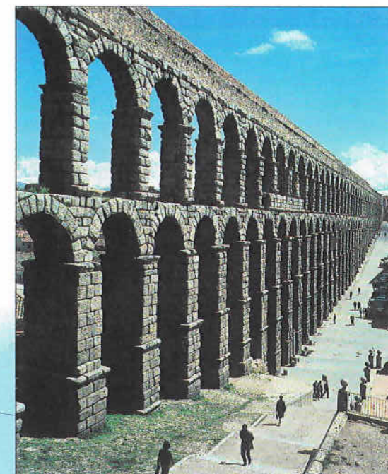
Right: the aqueduct at Segovia was probably built during the reign of Trajan. The great arches that tower 128 ft (39 metres) over the city are just the final section of a watercourse that starts in the hills 10 miles (16 km) away.
