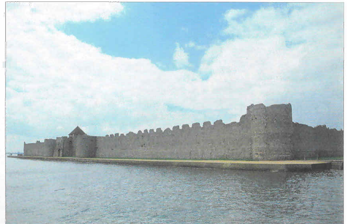
Below: Portchester Castle near Portsmouth is the best-preserved of the chain of coastal forts built on both sides of the English Channel in the late 3rd and early 4th centuries. The rounded projecting towers are typical of later Roman military architecture. In the 4th century this and the other coastal forts were placed under the command of a single military officer, the comes litoris Saxonici—Count of the Saxon Shore—whose job was to protect eastern Britain from the activities of Saxon pirates.
