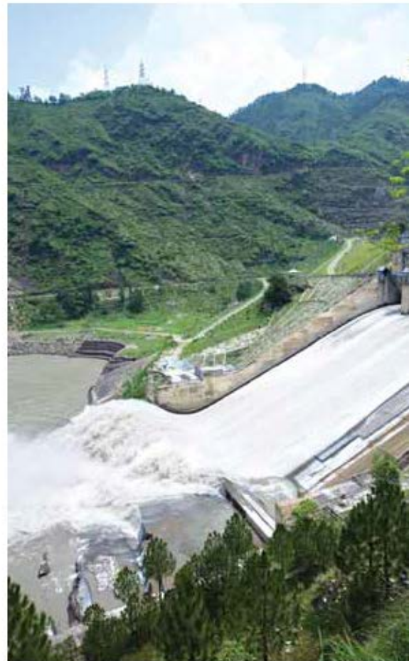
Pandoh Dam near Tandi in India. Hydroelectric power constitutes about a quarter of India's energy.
