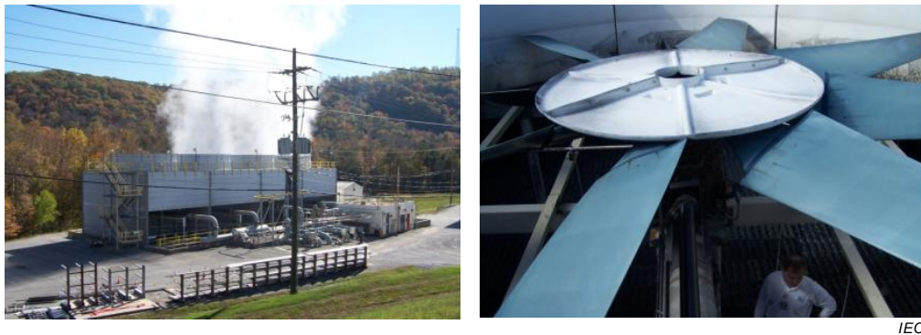
Figure 21 – Installation of permanent wireless monitoring system at ORNL HFIR cooling tower (8-2011)
