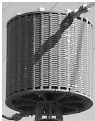
Figure 23 – Circuit-bouchon HT
