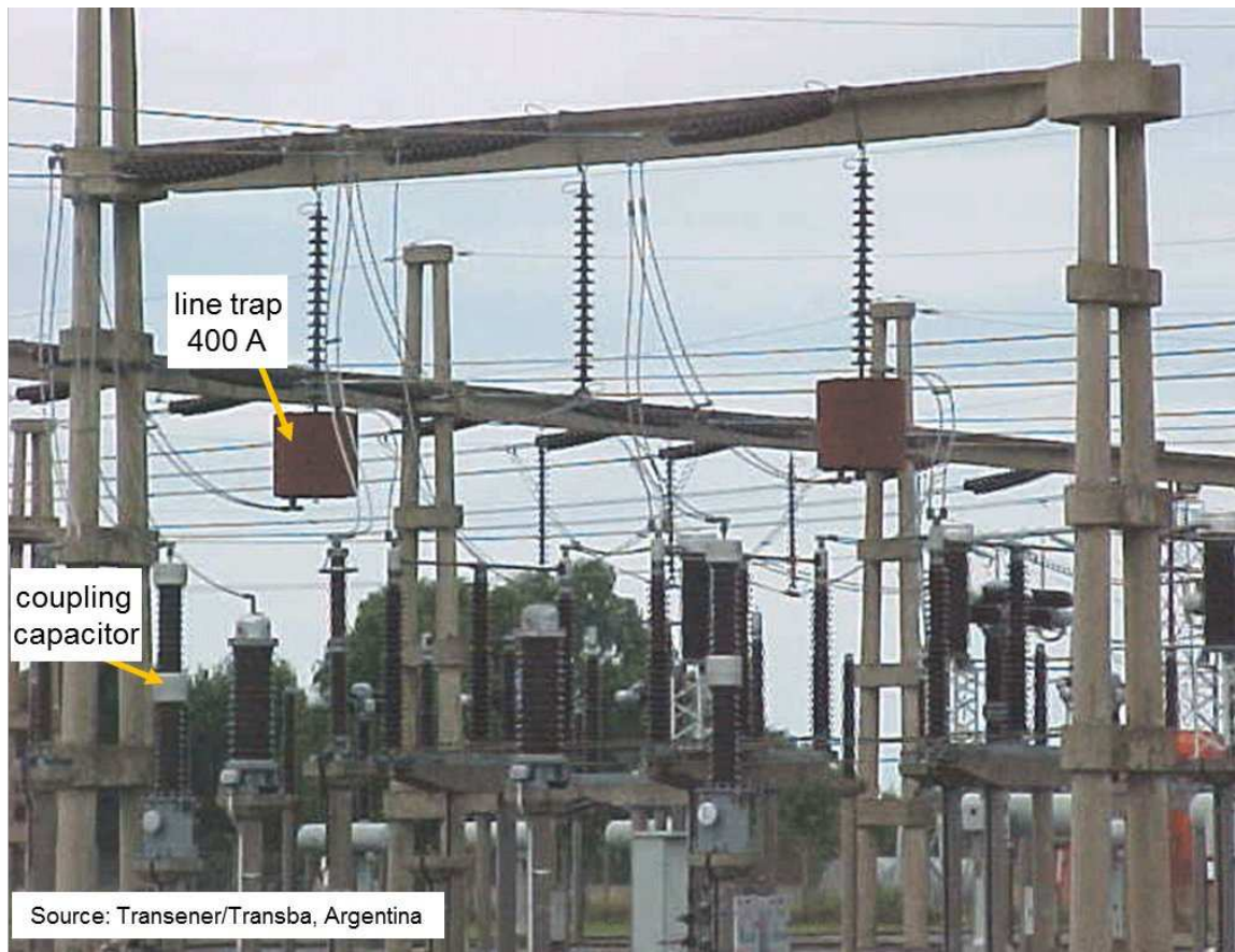
Figure 29 – Phase-to-phase signal coupling
