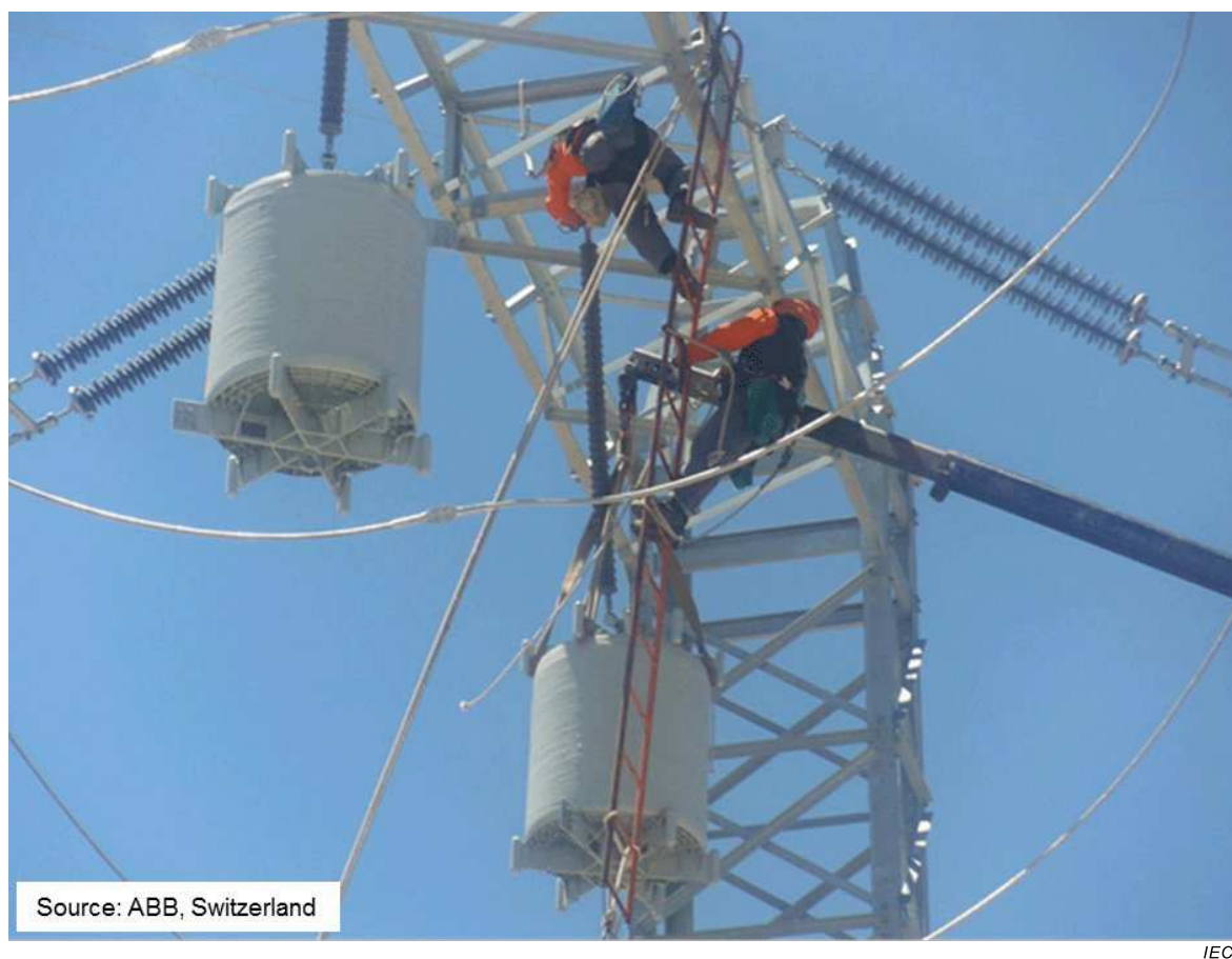
Figure 30 – Power line carrier, line traps
