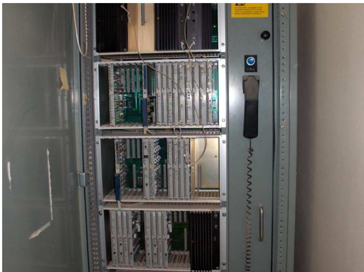
Figure 4 – Cabinet of the substation edge node
