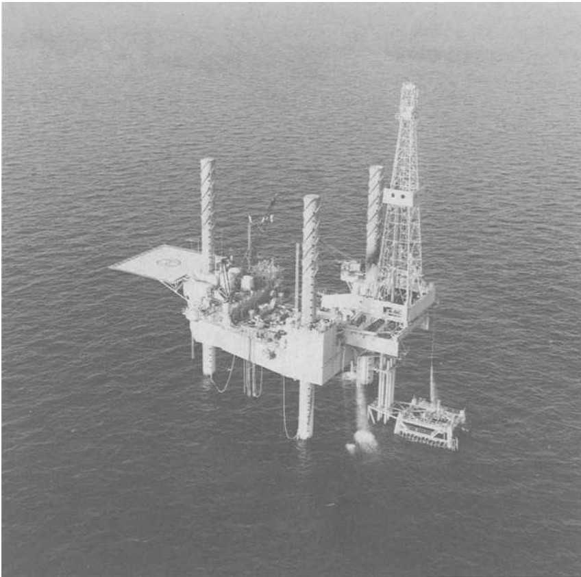
FIG 6—Scruton spoilers installed on jack-up rig legs.
