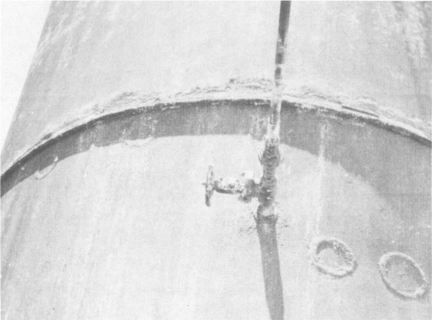
FIG. 3—Corrosion above an insulation support ring and around a small pipe connection. This is a vertical drum that had been heated with a steam coil at one time. Insulation rings act as a hold up for water entering through deficient top head weatherproofing.
