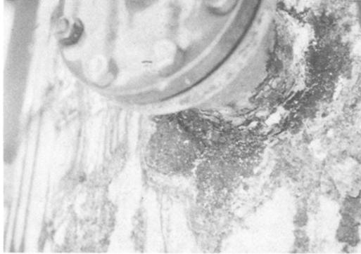
FIG. 2—Example of corrosion under insulation. This area is in the kettle section of a column, which was slightly above ambient. Upper portions of the column run well below ambient and condense moisture, which runs down the wall. The proper coating had been used, but it had been applied too thin. Pinholes allowed the corrosion to get started.
