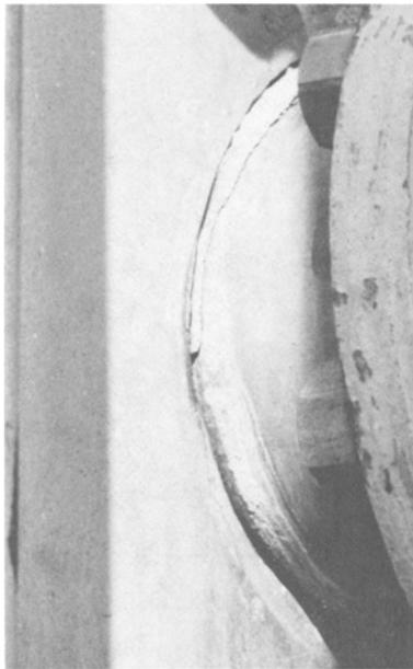
FIG. 1—*Deteriorated caulking, stainless steel vessel.*
