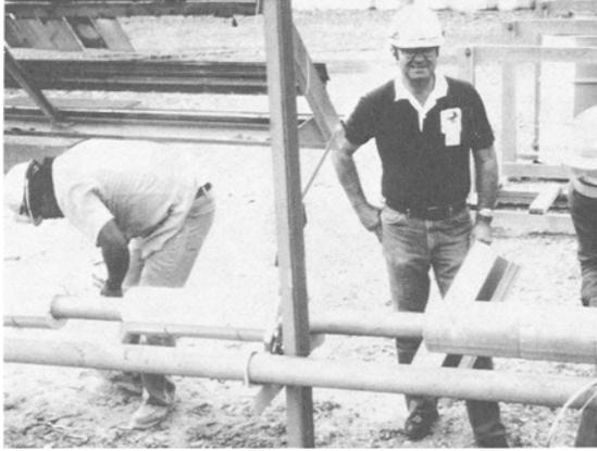
FIG. 5—Insulation being applied to the pipe by skilled insulators.
