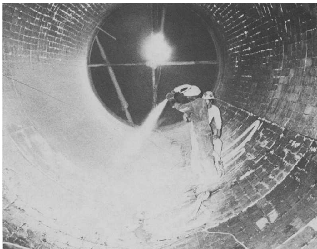
FIG. 7-6—Field installation of a cementitious monolithic being applied by pneumatic gun. (Photograph courtesy of Pennwalt Corporation, Corrosion Engineering Division.)
