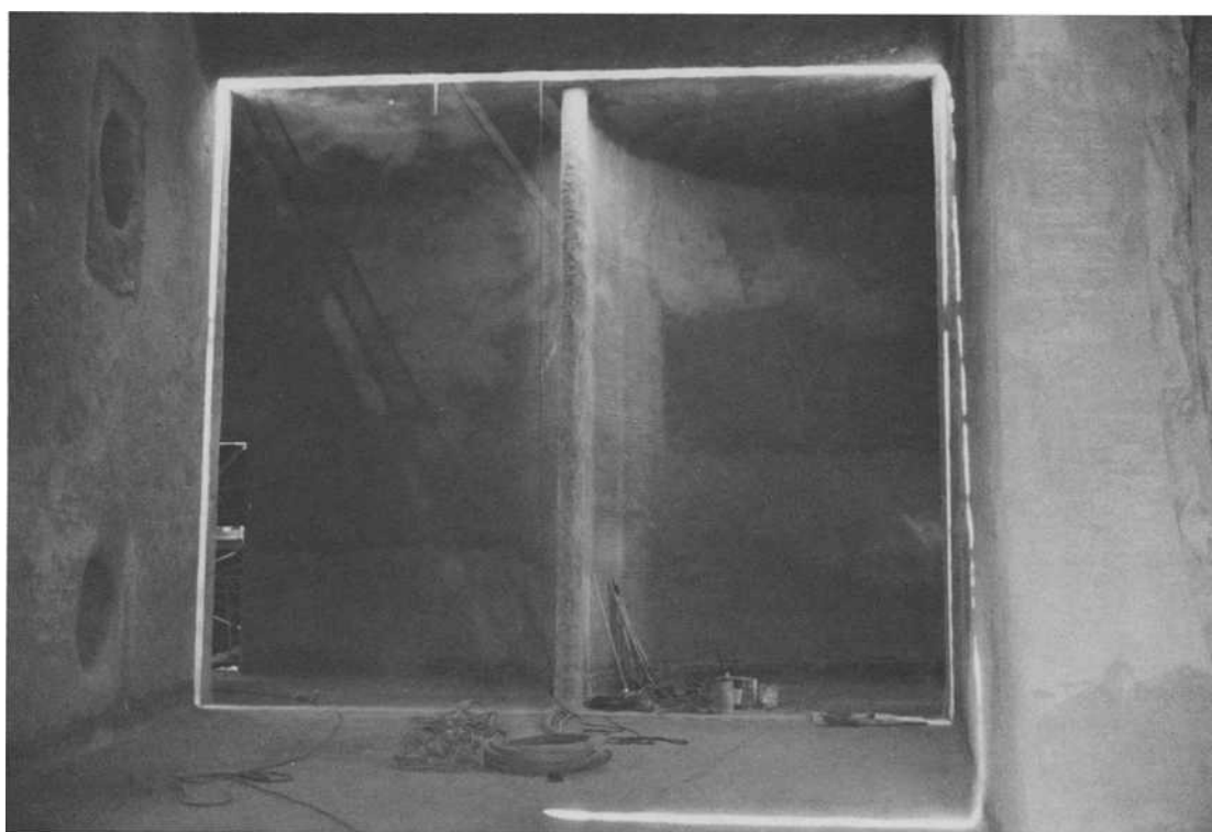
FIG. 2-5—Typical duct intersection, such as the by-pass duct intersecting the absorber outlet duct. (Photograph courtesy of Stone and Webster Engineering Corporation.)
