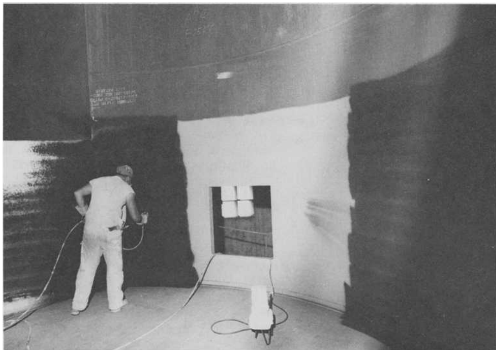
FIG. 7-2—Application of a liquid-applied fluoropolymer. (Photograph courtesy of Gilbert/Commonwealth.)
