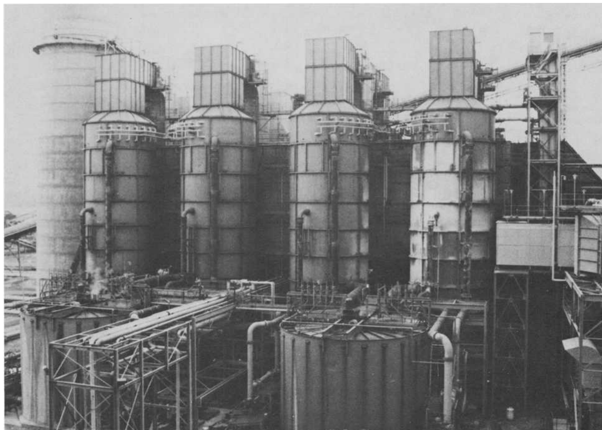
FIG. 1-1—General view of a limestone FGD system showing four of eight absorber towers. (Photograph courtesy of Stearns-Roger Engineering Corporation.)
