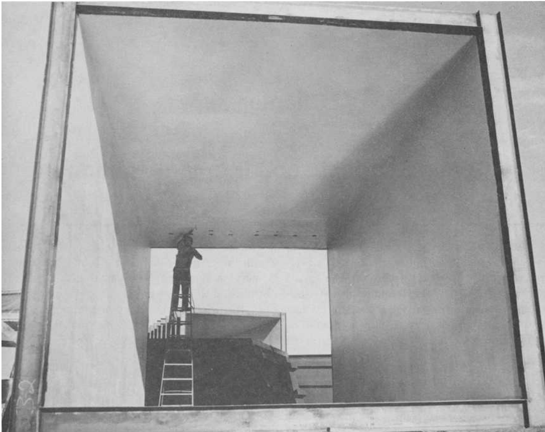
FIG. 3-1—Organic lining as applied in the field. (Photograph courtesy of Ceilcote Company, unit of General Signal.)
