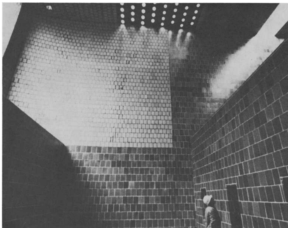
FIG. 3-5—Chemically resistant masonry construction used in FGD system. Lighter area is acid-resistant brick with furan resin; darker area is acid-resistant tile with vinyl ester resin. (Photograph courtesy of Stebbins Engineering and Manufacturing Company.)
