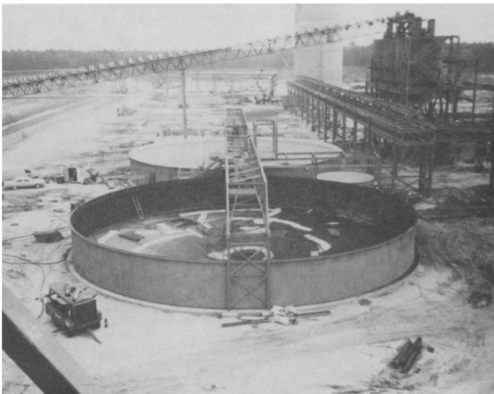
FIG. 1-5—Thickener tank for treating effluent from FGD system. This tank has a concrete bottom and steel side walls. (Photograph courtesy of Ceilcote Company, unit of General Signal.)
