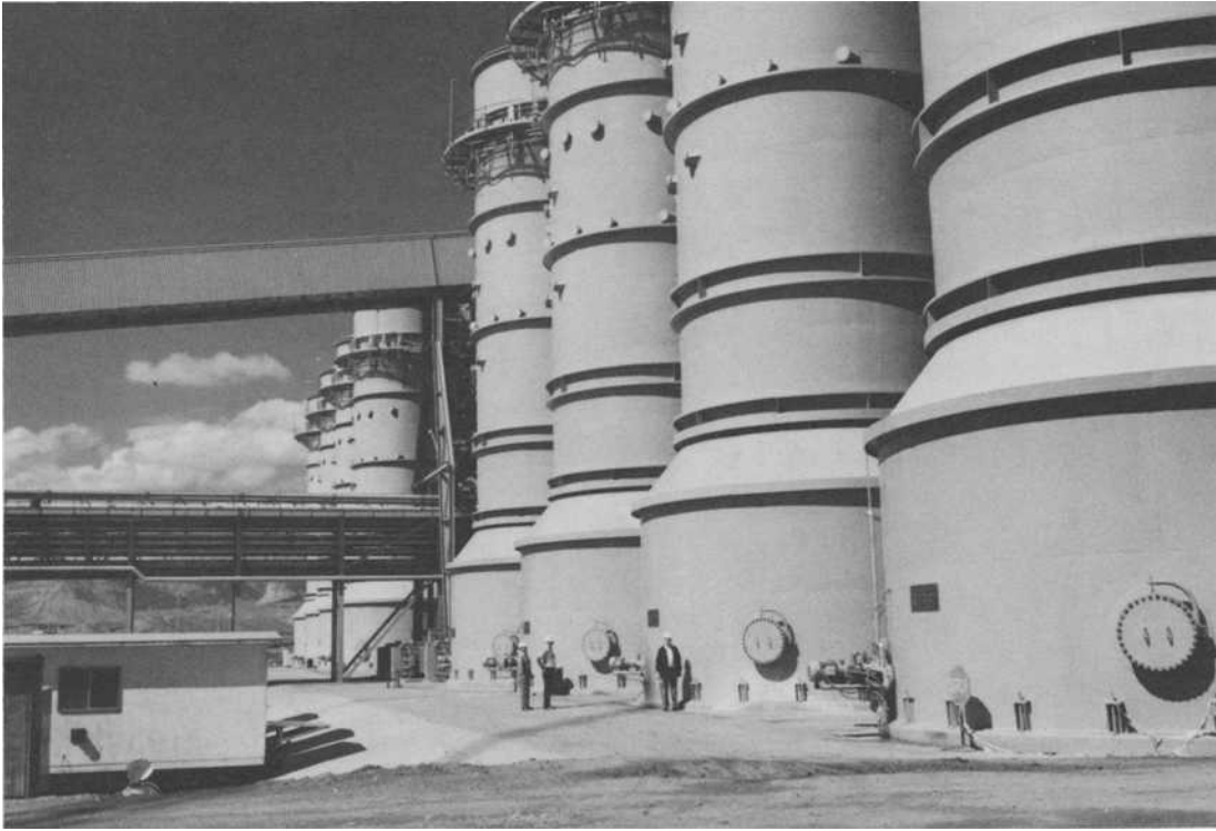
FIG. 1-2—Absorber towers of FGD system. (Photograph courtesy of Ceilcote Company, unit of General Signal.)
