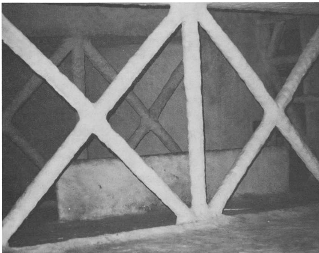
FIG. 3-3—Inorganic cementitious monolithic lining applied in mixing zone area over complex shapes and surfaces. An organic resin membrane is used under the inorganic material. (Photograph courtesy of Pennwalt Corporation, Corrosion Engineering Division.)
