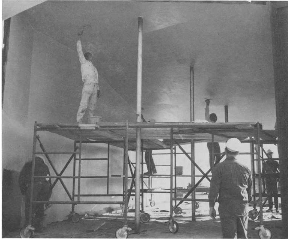
FIG. 7-1—Field application of organic linings. (Photograph courtesy of Ceilcote Company, unit of General Signal.)
