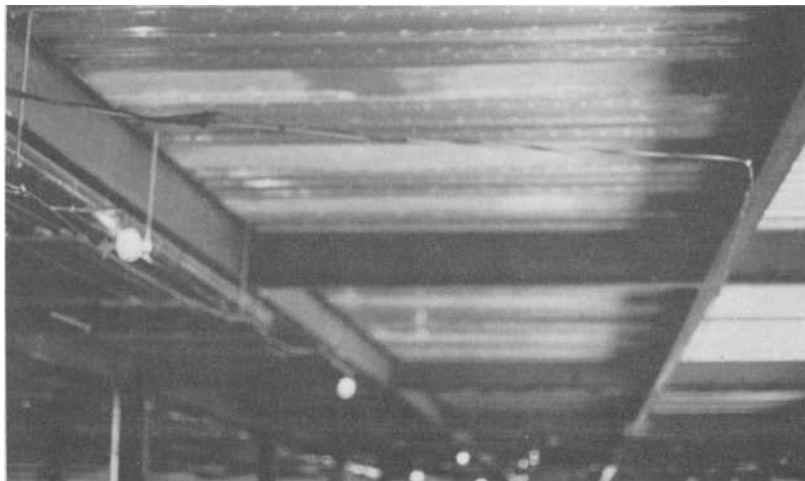
FIG. 5— Beam and deck construction ready for spraying.
