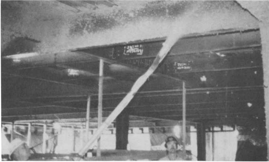
FIG. 5—Workers spray steel structural members with fire resistive material. Photo courtesy of the United States Mineral Products Co.
