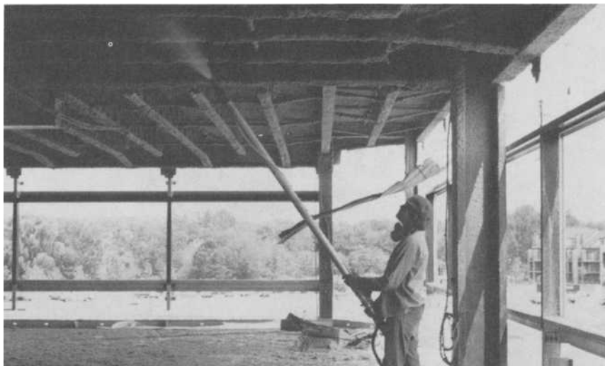
FIG. 4— Vertical spraying of mineral fiber composition using a pole gun.
