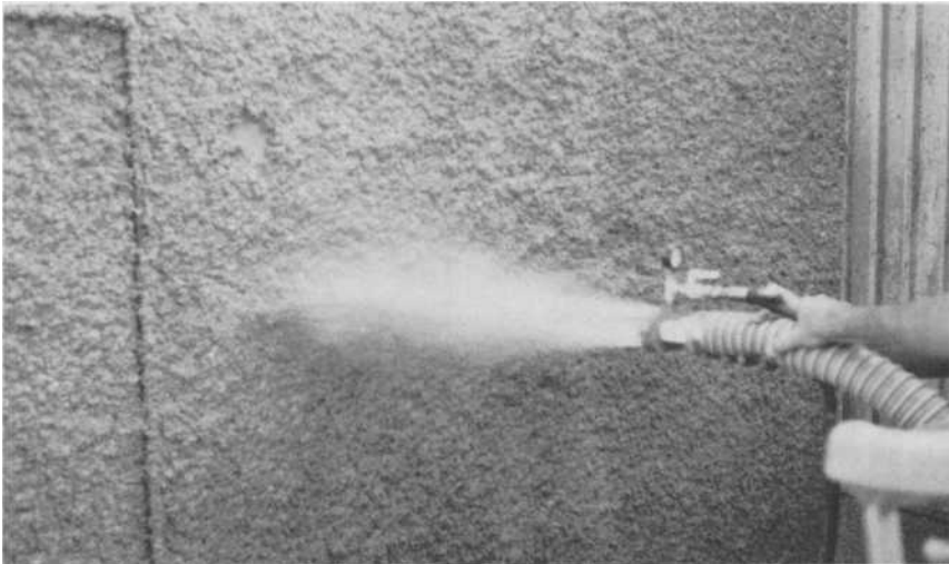
FIG. 3—Horizontal spraying of mineral fiber composition.
