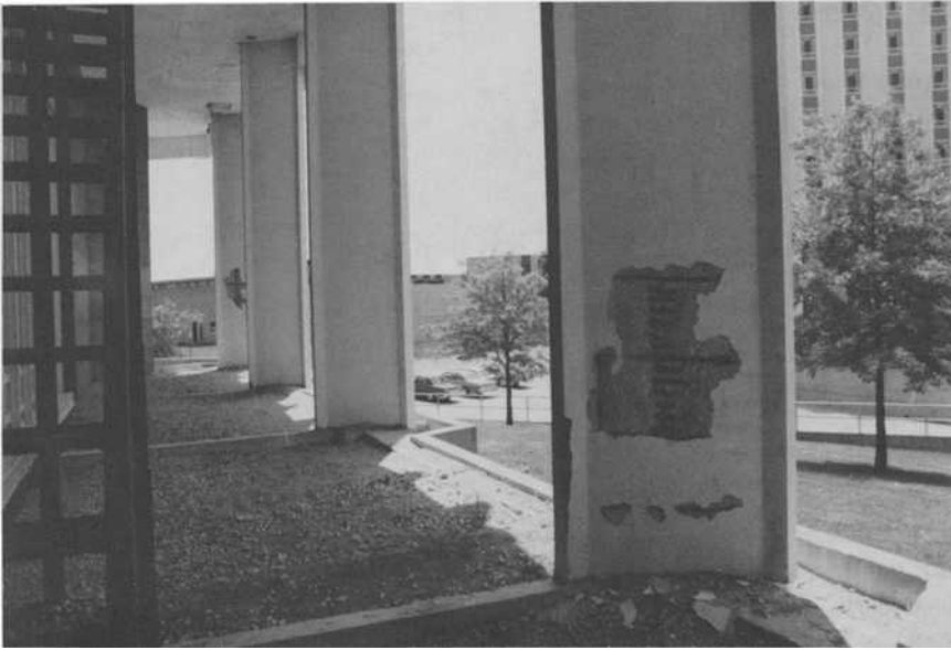
FIG. 5—Spalling on building columns due to chloride admixture and inadequate depth of cover.
