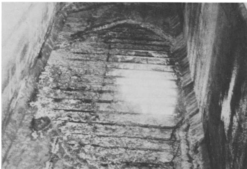
FIG. 2— Ultimate deterioration of bridge deck due to chloride corrosion of reinforcing steel.
