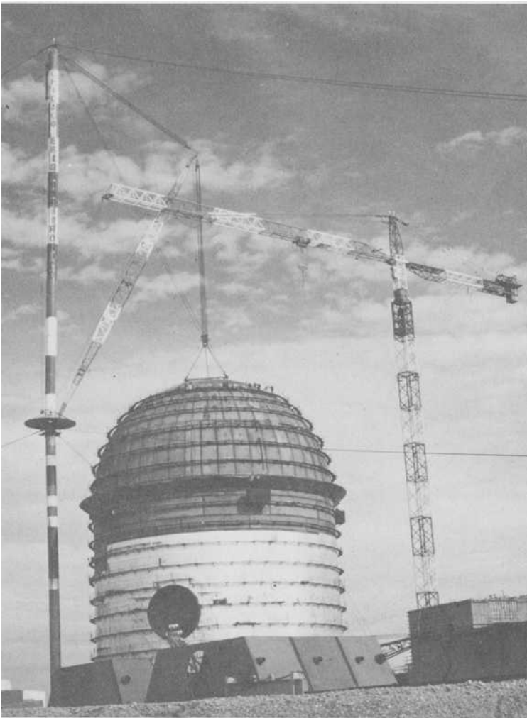
FIG. 8—Nuclear containment vessel being insulated for PWHT.
