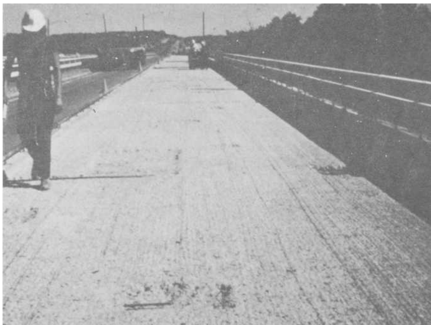
FIG. 3—Floor ready for resurfacing. Areas of unsound concrete removed and remaining concrete scarified.
