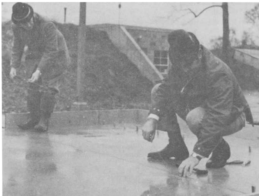
FIG. 12—Installation of the platinum-surfaced niobium wire anode into a groove cut in prototype bridge deck.
