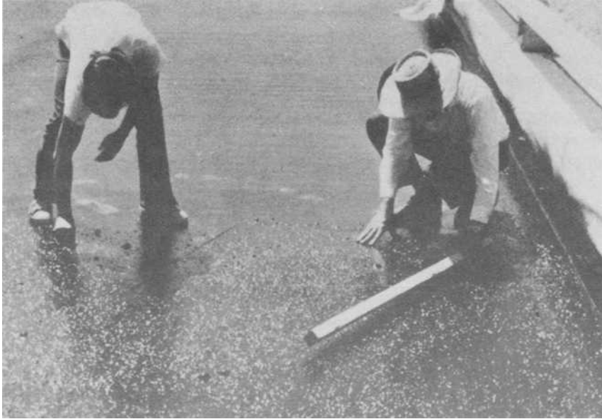
FIG. 2—Comparison of membrane sprayed over heated and unheated deck. Time: 9 to 9:30 a.m.
