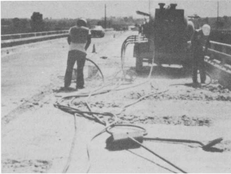
FIG. 1—Pneumatic hammers (#30 maximum) used in initial removal of unsound concrete.
