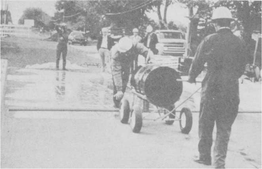
FIG. 2— Application of monomer during the partial impregnation of a cast-in-place bridge deck.
