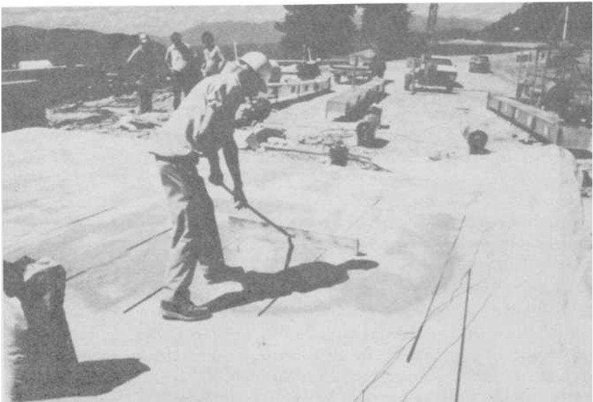
FIG. 3— Removal of sand layer after the partial impregnation of a cast-in-place bridge deck.
