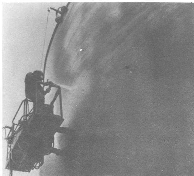
Figure 1. Mechanized, revolving scaffolds permit fast application of spray urethane foam insulation on refinery storage tanks.
