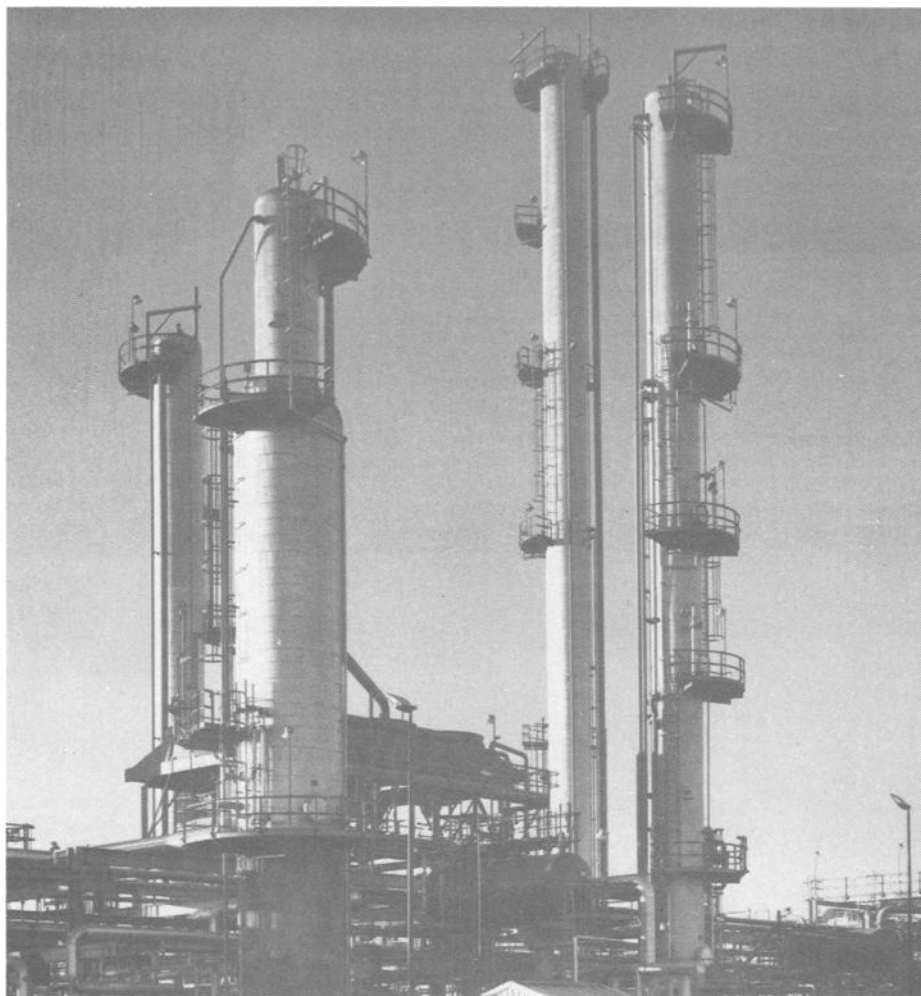
Catalytic cracker and alkylation unit at an oil refinery. All piping, vessels, tanks, and towers protected with 3/16-in. corrugated and deep-corrugated aluminum sheets.
