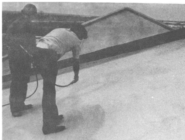
Figure 6. One-component silicone rubber coating being sprayed over a polyurethane foam.
