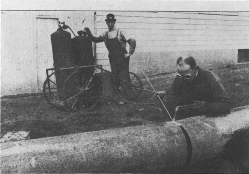
FIG. 1—1911 style of oxyacetylene welding.
