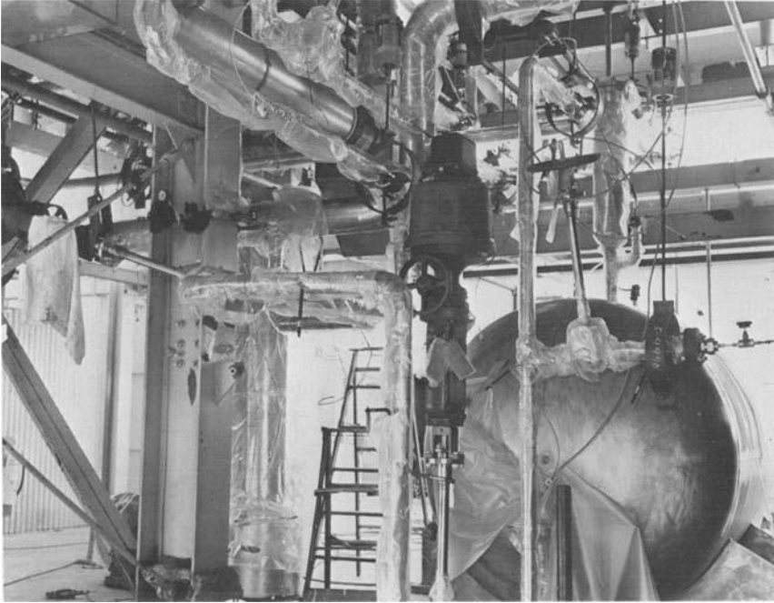
FIG. 2—Current precautions being taken to protect stainless steel surfaces during construction of liquid metal heat transport systems.
