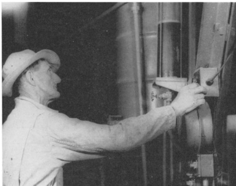
FIG. 2.—Admixture Dispenser Showing the Calibrated Sight Glass.
