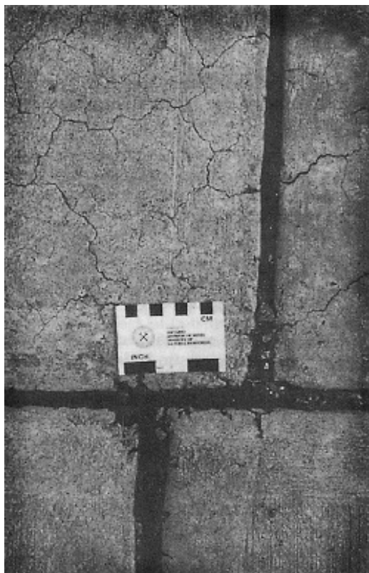
Fig. 2 —Concrete slab affected by alkali-carbonate reaction (upper portion of photo) that has moved 9 cm to the right relative to the concrete in the lower portion of the photo that has nonreactive aggregate. Expansion was measured at 1.2 % in three years, Ontario, Canada [48].
