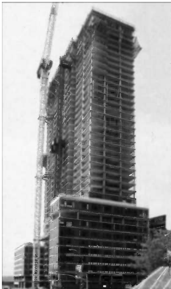
Fig. 21 —Forty-five percent slag cement concrete was used in the structural concrete in The Helena, in Manhattan, to help gain green building certification and a New York State tax incentive for green building construction. Two-day forming cycle was not affected by the use of slag cement, even though much of the construction occurred during the winter.
