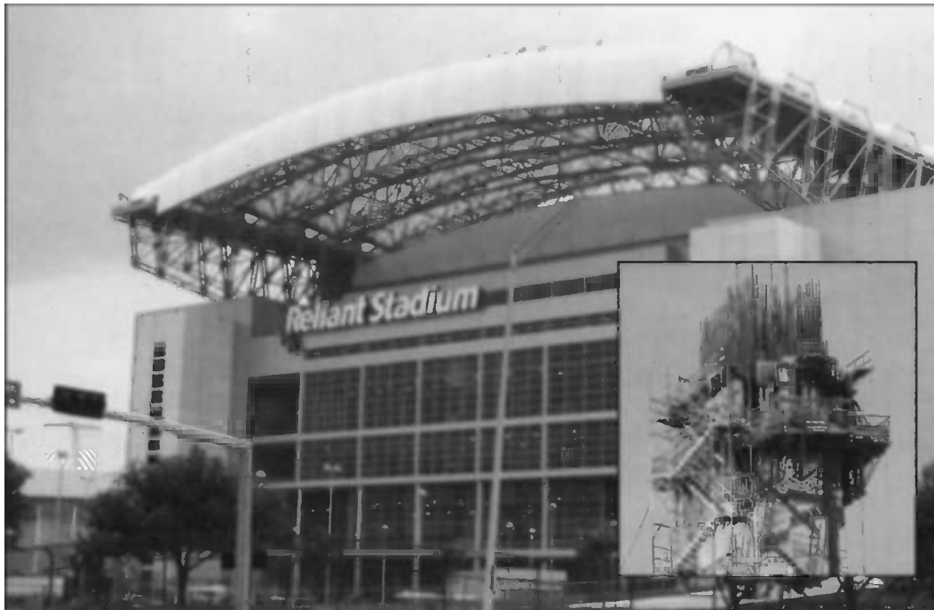
Fig. 20 —Reliant Stadium in Houston, home of the NFL Texans, utilized a high-performance ternary mixture of portland and slag cements and Class C fly ash in the four massive “super columns” that support the retractable roof (inset). The concrete met the requirements of high strength (13 000 psi), low heat (massive placement), and virtually self-consolidating consistency.
