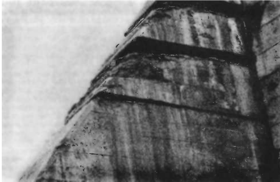
Fig. 16 —Deterioration at top of lifts in a dam from which the porous-nondurable concrete was not adequately removed prior to sequential lift placement. The poor quality concrete at the lift surface was caused by excessive bleeding and deteriorated due to frost action.
