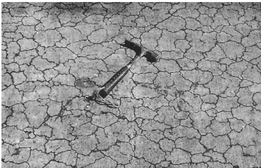
Fig. 1 —Typical cracking of concrete slab by alkali-carbonate reaction after three years, Ontario, Canada [7].
