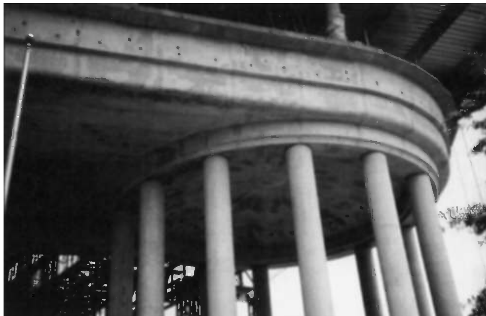
Fig. 19 —Greening is evident after forms were removed from the Canadian Embassy in Washington, DC. Greening disappeared after several weeks resulting in the desired light concrete appearance of slag cement concrete (see Fig. 17).
