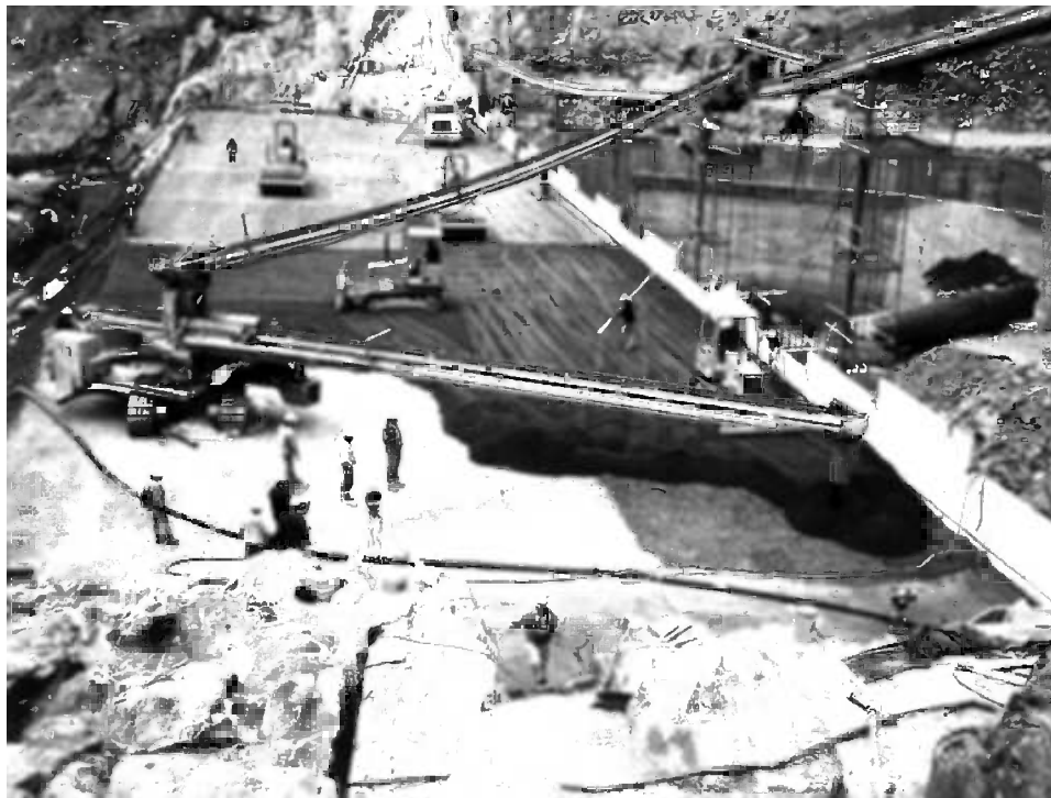
Fig. 1—Construction of C. E. Siegrist Dam, PA. Note use of conveyors to place roller-compacted concrete (photo courtesy of Gannett Fleming).
