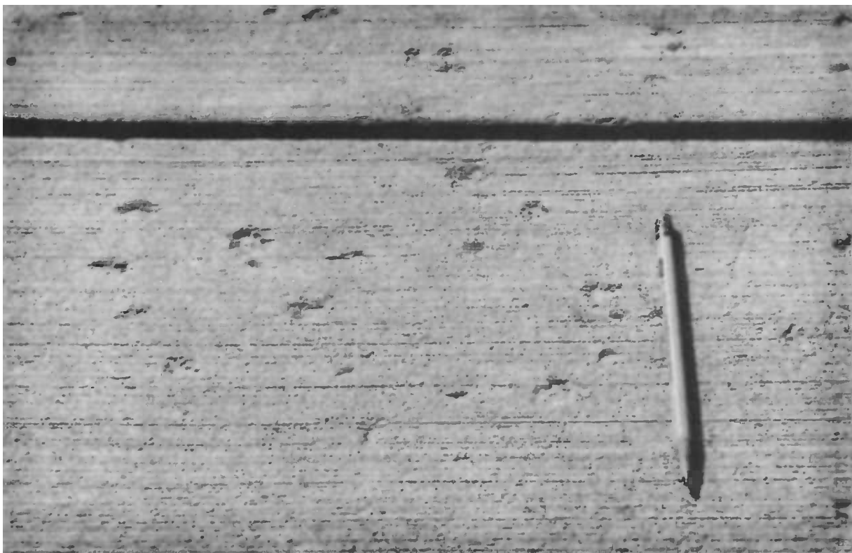
Fig. 19—Mortar flaking over coarse aggregate (photo courtesy of the Portland Cement Association).
