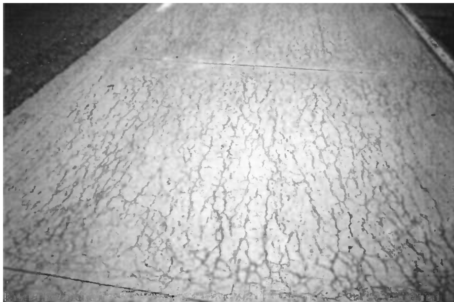
Fig. 2 —Longitudinal cracking initiated by ASR in a jointed, slab-on-grade pavement. A longitudinal crack pattern prevails in this pavement, together with minor random cracking, particularly near transverse joints.
