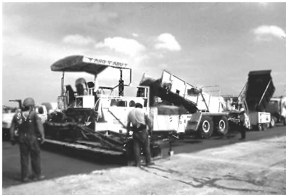
Fig. 2 —RCC being placed with heavy-duty paver. Intermediate transfer device used to maintain a constant flow of material to the paver.
