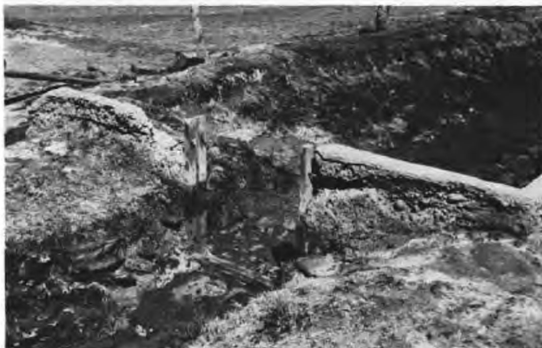
FIG. 5—Concrete under ground was intact, but rising sulfate solutions caused exposed surfaces to spall away as salt crystals developed in concrete pores as moisture evaporated.
