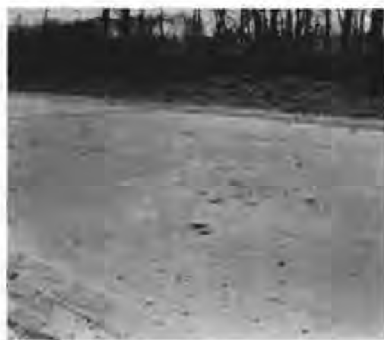
FIG. 1—Popouts produced by claystone, shale, and chert in concrete pavement near Jackson, Mich.
