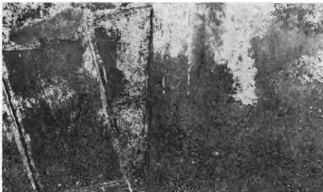
FIG. 1—Lime-hungry or slightly acid water has leached surface mortar and exposed small aggregate on surfaces of this siphon inlet.
