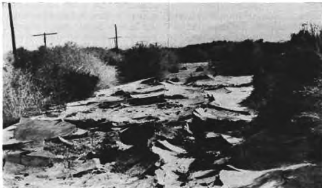
FIG. 3—This World War II air base barrack floor in a desert location showed distress in a few years from sulfate attack.
