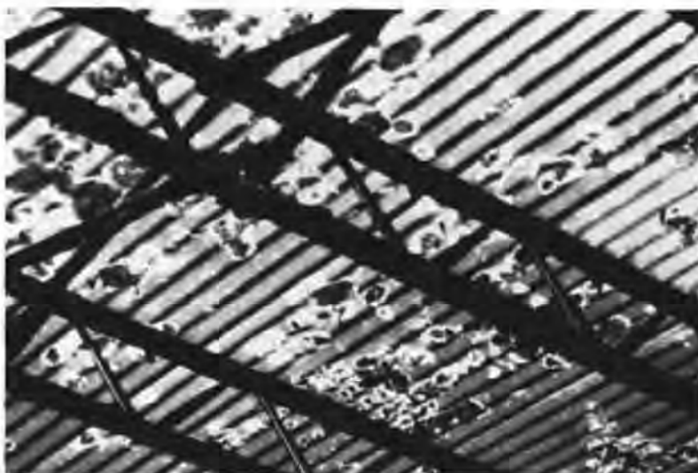
FIG. 3—Corrosion and perforation of galvanized steel from under concrete slab (from Ref. 10)
