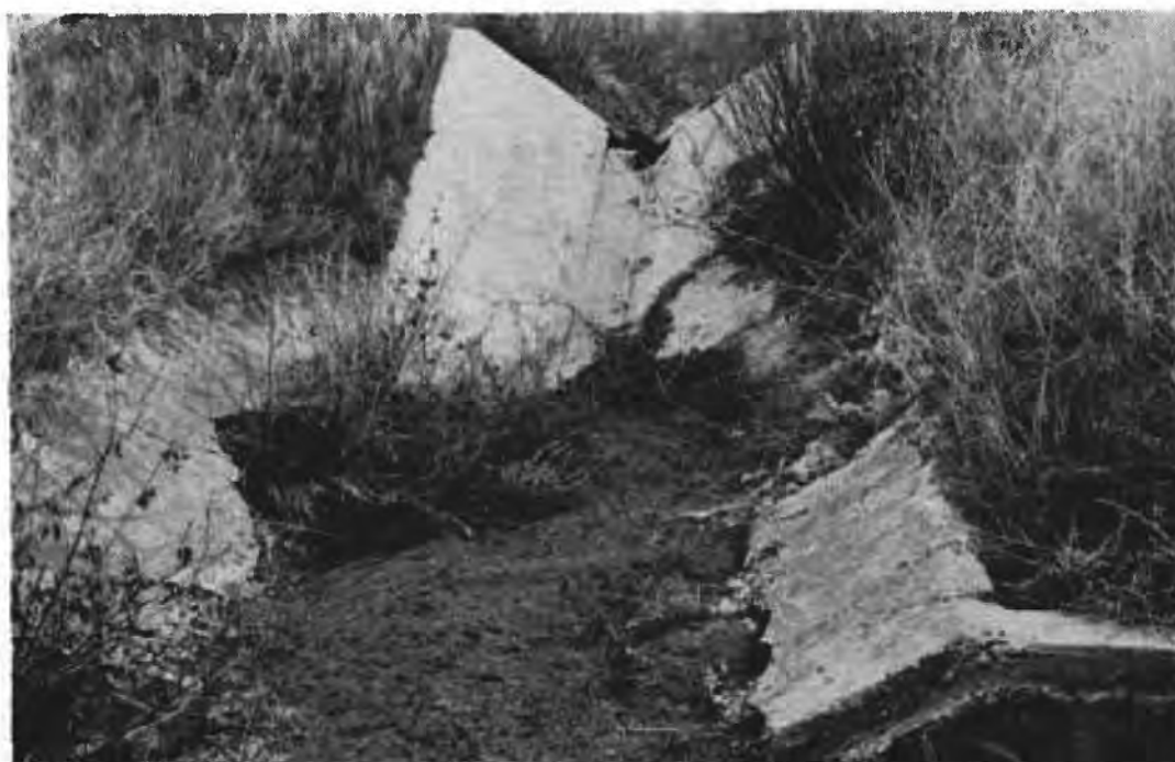
FIG. 4—Corrosion by sulfates has completely disintegrated lower parts of this drop structure in a western canal.
