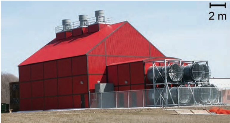
FIG. 1—Univ. of Waterloo Live Fire Research Facility.
