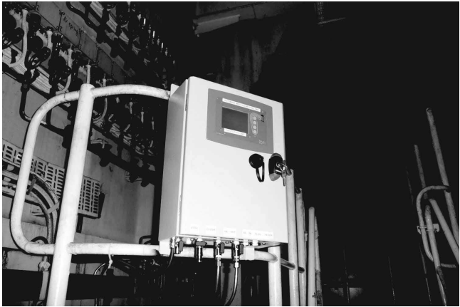
FIG. 12— Slow speed diesel engine installation.
