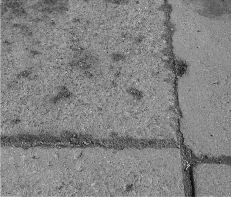
FIG. 3—*Severely scaled sidewalk.*
