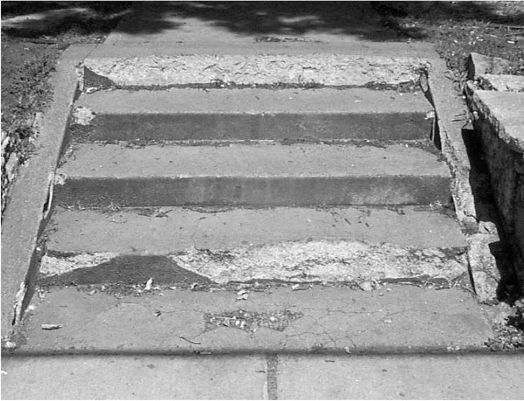
FIG. 1—Loss of concrete from stairs due to internal freeze-thaw damage.
