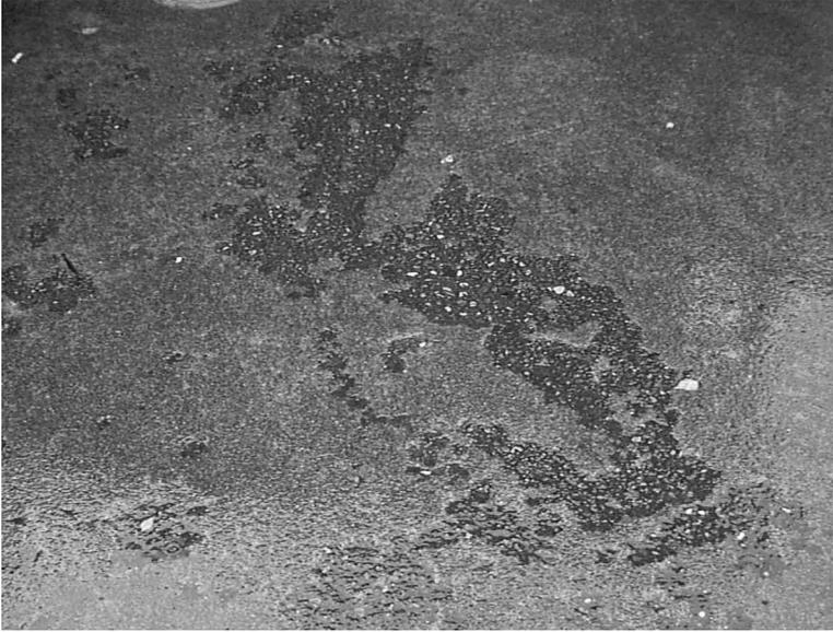
FIG. 4—*Significant variation in surface scaling.*
