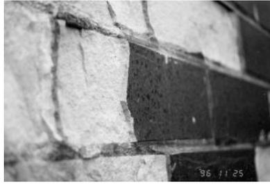
FIG. 5—Cryptofluorescence behind the spalling faces of the glazed brick.
