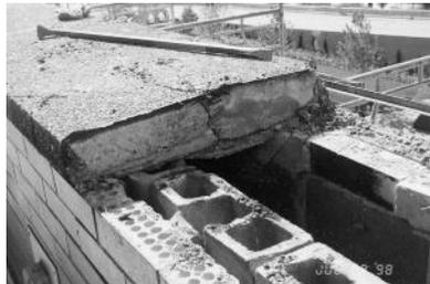
FIG. 7—Original concrete coping with surface cracks. No through-wall flashing was found below the coping.
