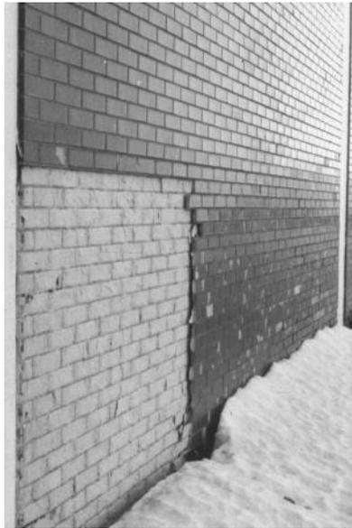
FIG. 1—Spalling of the faces of glazed brick caused by freeze/thaw action.
