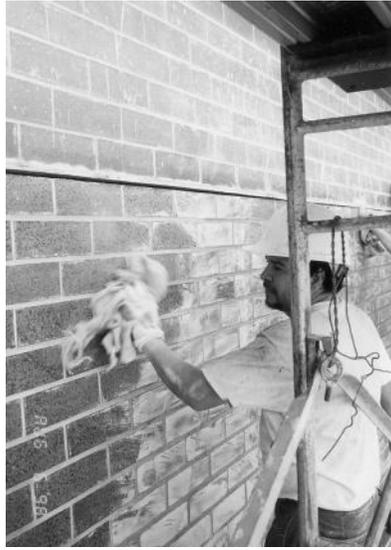
FIG. 11—*Removal of excess grout from the glazed brick after grouting of the mortar joints.*
