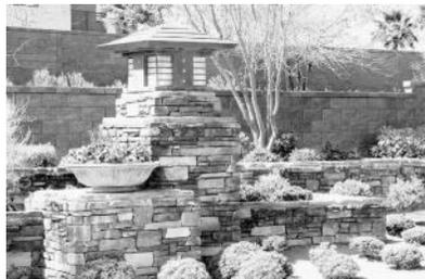
FIG. 1—Adhered veneer on concrete block retaining walls. (Red Rock Country Club; Las Vegas, Nevada. Photo by R.J.Godbey.)
