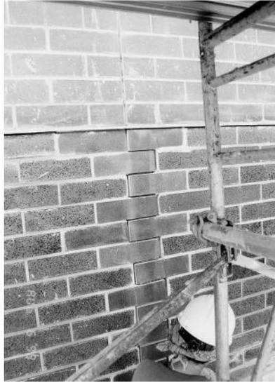
FIG. 10—*Ineffective portions of the stepped expansion joints were rebuilt. The vertical expansion joints in the parapet wall above are straight instead of stopped.*
