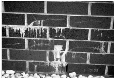
FIG. 4—Efflorescence present on the face of the glazed brick at mortar joints and cracks.
