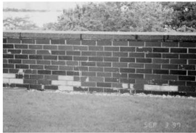
FIG. 3—Existing parapet wall exhibiting significant spalling and cracking of the faces of the glazed brick.
