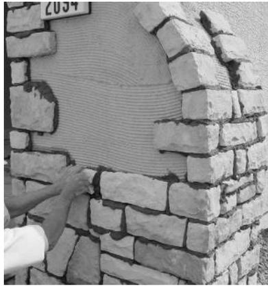
FIG. 2—Backing prepared with horizontally raked stucco scratch coat, layout completed, corner stones set, adhered veneer installation proceeding. (Summerlin Masterplanned Community; Las Vegas, Nevada. Photo by R.J. Godbey.)
