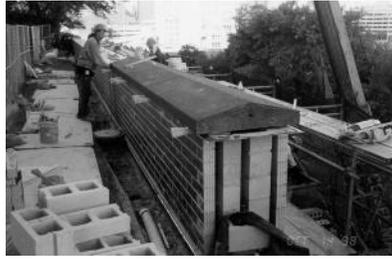
FIG. 9—The new parapet wall with through-wall flashing below the coping and 2-in. wide drainage and ventilation cavities.
