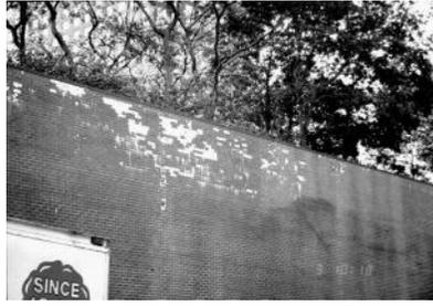
FIG. 2—Existing parapet wall and portions of the top of the wall below the parapet exhibiting significant spalling and cracking of the faces of the glazed brick.
