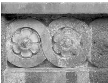
FIG. 5—Detail of a cast Roman cement element after uncovering from a layer of cement spray mortar; such work is time consuming if carefully executed and would therefore be performed only exceptionally.
