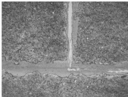
FIG. 5—Close-up view of original natural cement pointing mortar at Cheshire Mill No. 1, west elevation, showing ruled and penciled detailing.
