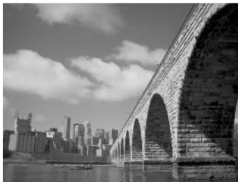
FIG. 6—The Stone Arch Bridge in Minneapolis is one of the numerous surviving structures documented as having been built with natural cement. Photo by the author.
