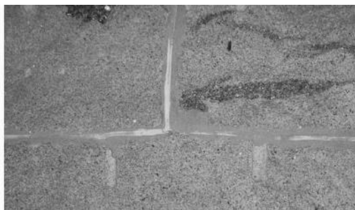
FIG. 13— Close-up view of ruled and penciled pointing details at Frost Free Library—Marlborough, New Hampshire.
