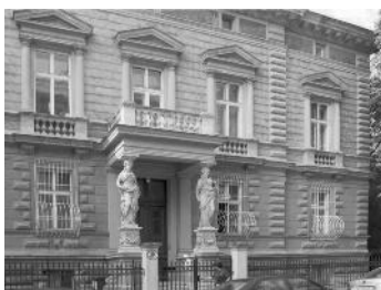
FIG. 2— Facade dating 1878 with light-brown Roman cement stuccoes covering the ground floor; Vienna, Austria. This is one of a few examples of a surface that was never painted.
