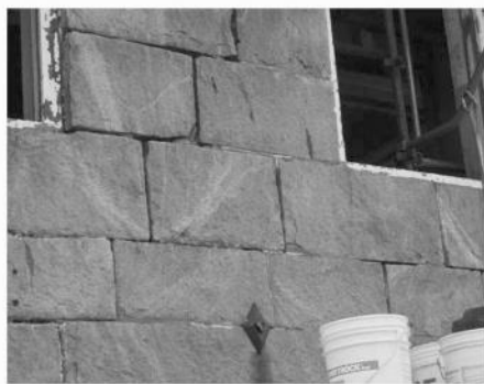
FIG. 7—Removal of incompatible portland cement repointing materials and unsound original mortars was performed prior to repointing with natural cement mortar.
