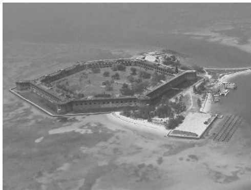
FIG. 1—Fort Jefferson, Dry Tortugas, Florida, offered 19th century engineers no fresh water for mixing of mortar and concrete. Seawater was used to no apparent detrimental effect. (Photograph courtesy of Michael Edison, 2004.)
