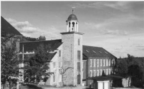
FIG. 3— Cheshire Mill No. 1, south elevation.
