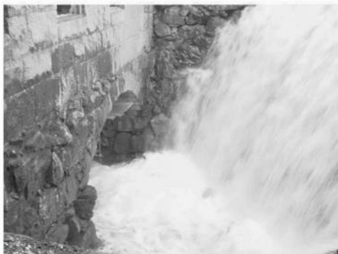
FIG. 6—Granite culvert spanning the river at Cheshire Mill No. 1, west elevation.
