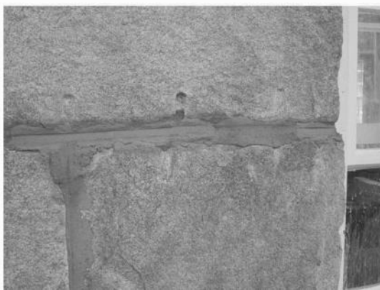
FIG. 16— Natural cement repointing mortar, after ruling.
