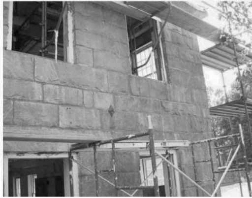
FIG. 17— Completed section of repointing.
