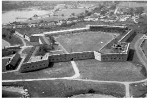
FIG. 2—Fort Adams, Newport, RI, was constructed from 1825–1838 using natural cement mortar, concrete, and stucco. Despite the lack of expansion joints and annual temperature ranges of over 55^{\circ}\text{C} ( 100^{\circ}\text{Fahrenheit} ), the structure exhibits no pattern of thermal expansion-related cracking or distress.
