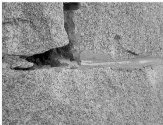
FIG. 9—Close-up view of prepared joint showing the extension of the lime bedding mortar nearly all the way to the surface of the joint.
