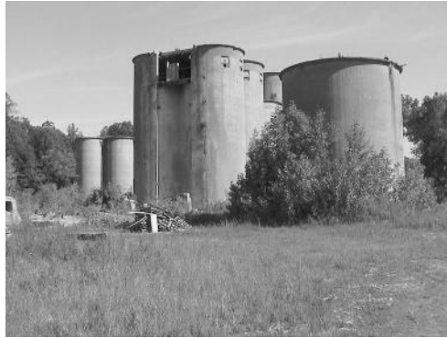
FIG. 5—Remains of the former Century Cement Company plant in Rosendale, NY, last of the original natural cement producers in the United States, closed in 1970. Natural cement mining in Rosendale was restarted in 2004 for production of natural cement for use in historic restoration. (Photograph Courtesy of Michael Edison, 2004.)
