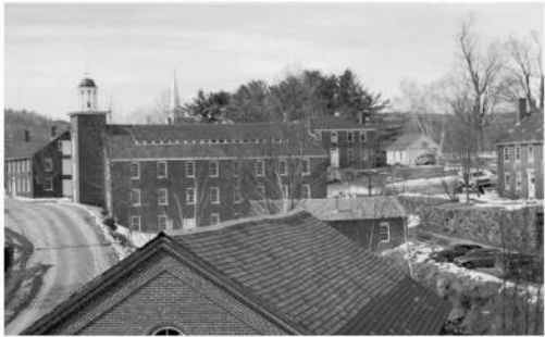
FIG. 2— Cheshire Mill No. 1, east elevation.
