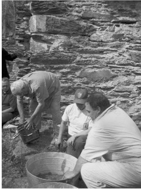
FIG. 7— Natural cement stucco preparation and application was demonstrated by masons from the National Park Service Historic Preservation Training Center at the Harper's Ferry pulp mill ruins during the Second American Natural Cement Conference. Photo by the author.
