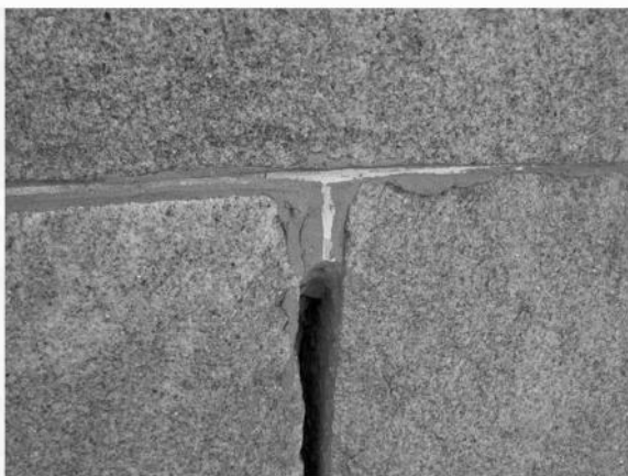
FIG. 10— Typical vertical joint prepared for repointing.
