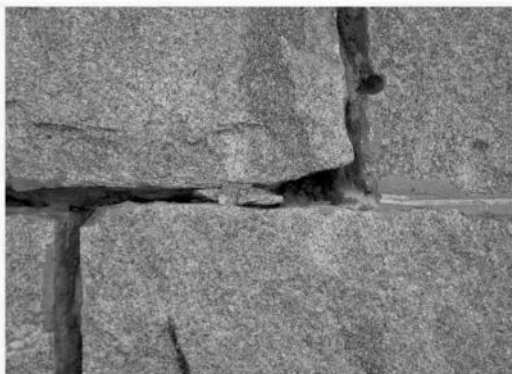
FIG. 8—Close-up view of prepared joint showing retention of original pin stones used in the stone-setting process.
