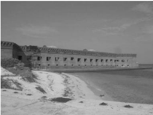
FIG. 2—Fort Jefferson’s remote location left 19th century engineers little choice but to make use of the excessively coarse calcareous beach sand that was at hand. (Photograph courtesy of Kenneth Uracius, 2004.)
