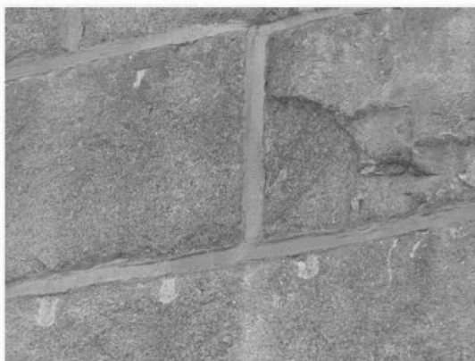
FIG. 11— Joint filled with Rosendale cement pointing mortar prior to detailing.
