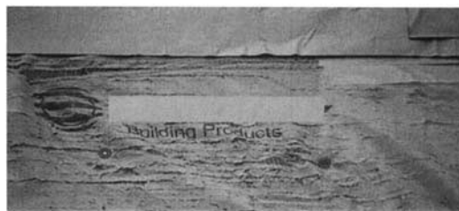
FIG. 18— Cracked and delaminated housewrap.
