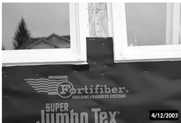
FIG. 17— Reverse lapped installation with no caulk.
