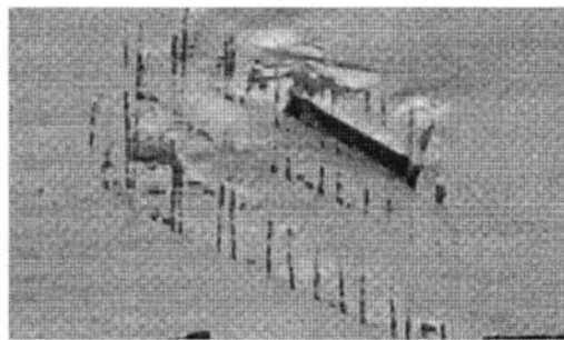
FIG. 13— Abrasive damage to weather resistive barrier from slap stapler.
