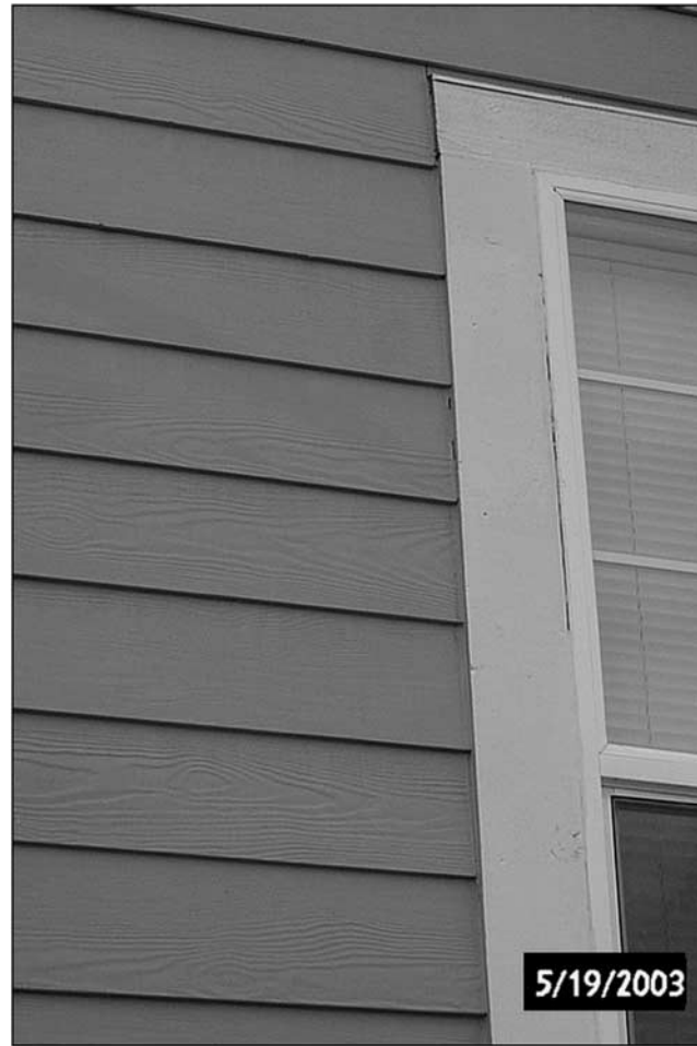
FIG. 30— Typical caulk failure at wood trim.
