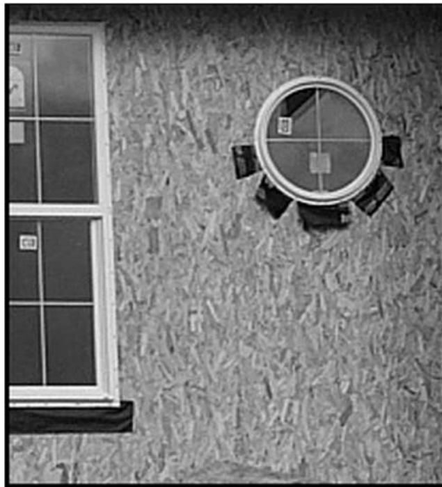
FIG. 19— A lack of basic flashing understanding.
