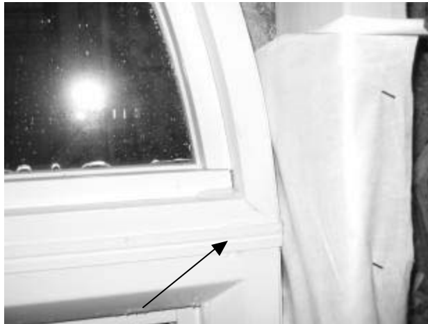
FIG. 16—Glazing leak in the vinyl clad round top window above the mullion to the vinyl clad square picture window.
