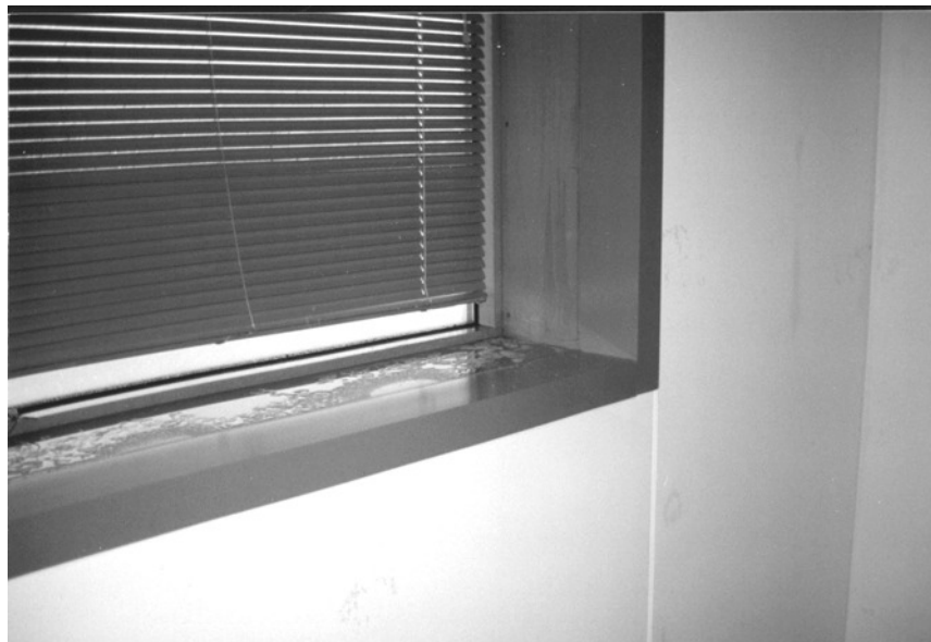
FIG. 11— Pooling of water at the stool.
