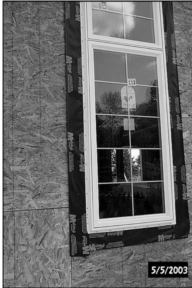
FIG. 23— Representative of many installations with no caulk.
