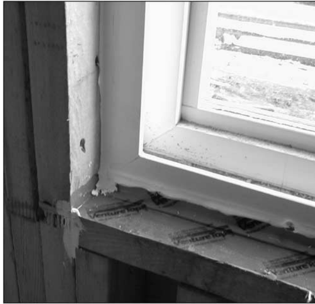
FIG. 9—A demonstration of installation of interior caulk.
