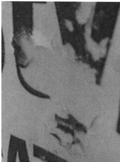
FIG. 14— Weather resistive barrier film damage.
