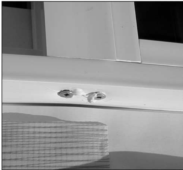
FIG. 27— Bolts neither tightened nor caulked adequately.
