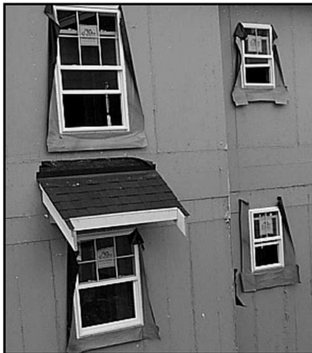
FIG. 14— Adhesive tape failure due to moisture.
