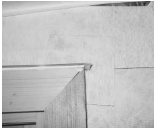
FIG. 2—Chevron made of nonwoven composite flashing installed at the corner of the head of a wood framed brick mold window.
