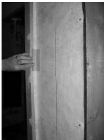
FIG. 6— Vinyl cladding details must conceal flashing details along the jambs of the brick mold window for the 90° turn method.
