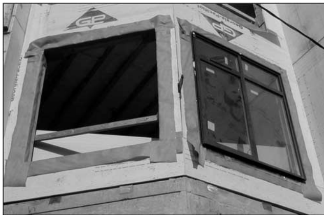
FIG. 7—Material designed as a roofing underlayment but used as flashing.
