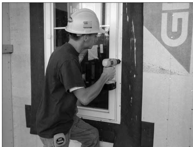
FIG. 15— An installer securing window with lathe screws.
