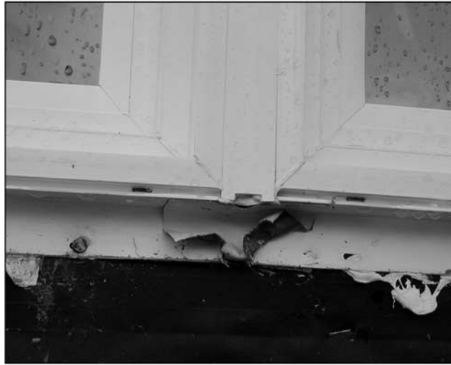
FIG. 28— Manufacture sealing tape failure.
