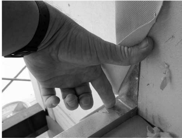
FIG. 13— Demonstration of metal sill pan.
