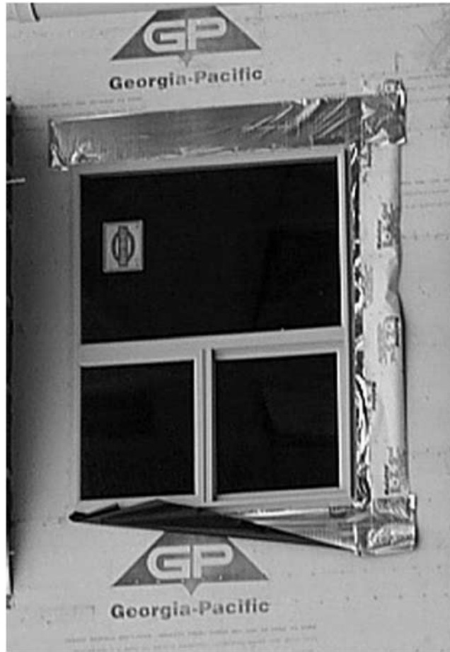
FIG. 5—A product with a fiberglass scrim bonded over gypsum.
