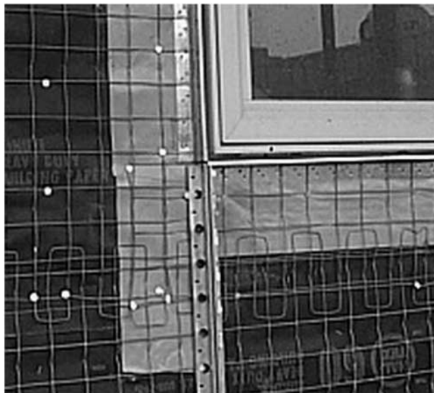
FIG. 31—A window prepared for stucco installation.
