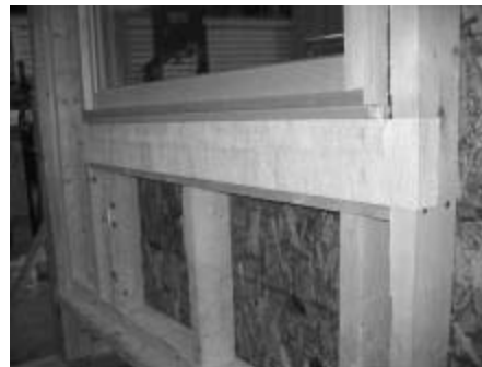
FIG. 10— Self-adhered flashing used to create an airtight seal between the top of the back dam and the interior sill of the window.
