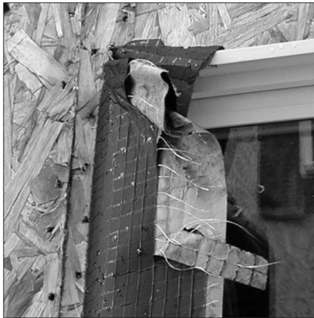
FIG. 29— Flashing that failed due to water and wind exposure.
