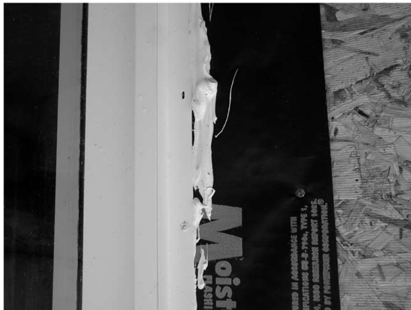
FIG. 16— Poor use of a lot of caulk in single family construction.
