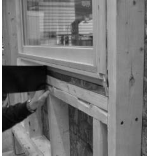
FIG. 9— Self-adhered flashing being applied to create an airtight seal between the top of the back dam and the interior sill of the brick mold window.
