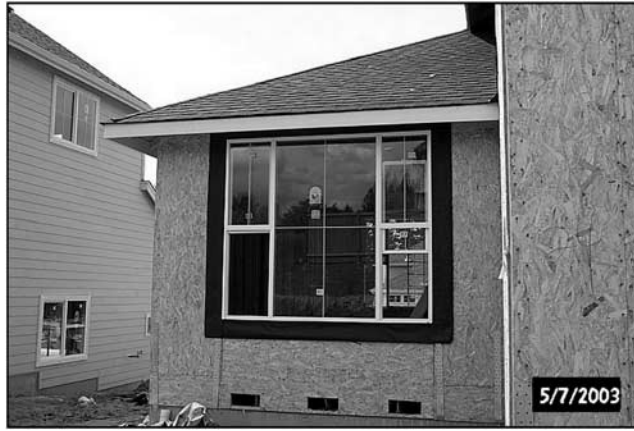
FIG. 25—Installation of a new gasket seal product.
