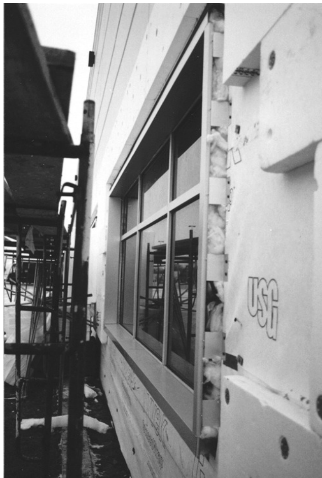
FIG. 13—Repair with exterior insulation and finish system and insulated frame covers.
