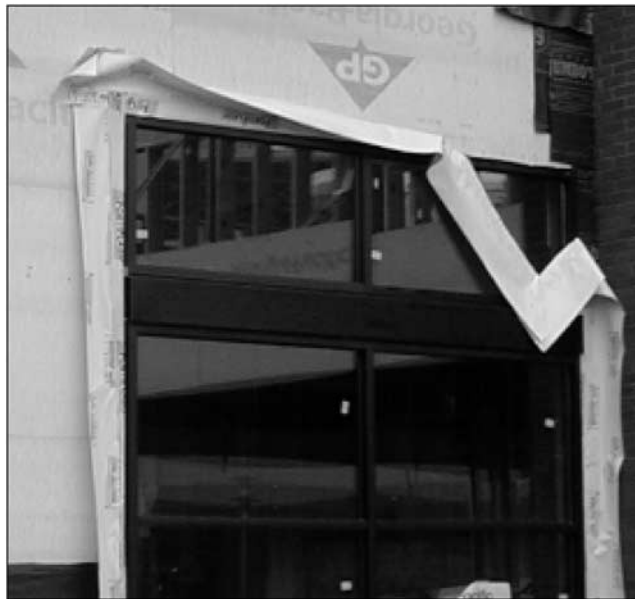
FIG. 21—Too few fasteners at head with little caulk.
