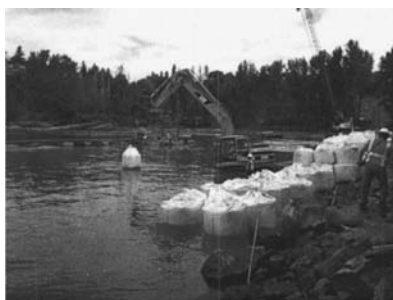
FIG. 1— Deployment of Organoclay Cap at Willamette River.
