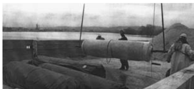
FIG. 3—Reactive material mat being prepared for deployment on the Anacostia River.
