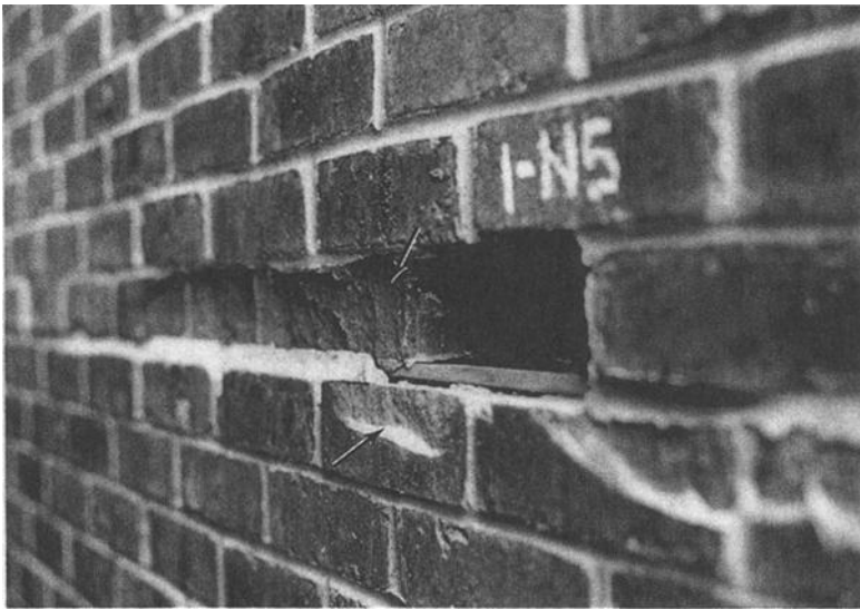
Figure 9--View of spalled brick due to compressive forces at shelf angle
