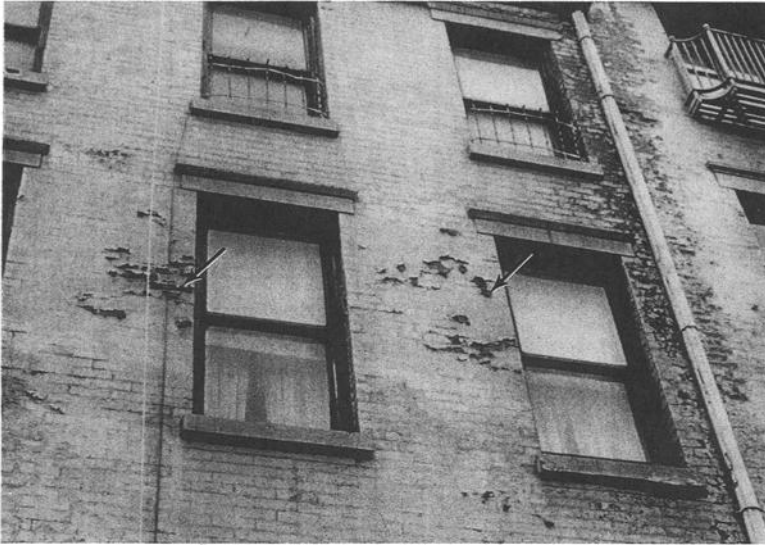
Figure 7--View of spalled brick due to cyclic freezing of moisture trapped by paint on brick
