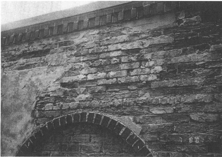
Figure 8 - View of spalled brick due to cyclic freezing of moisture and to cyptoflorescence behind stucco coating on brickwork
