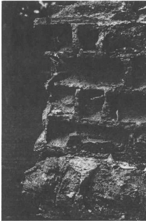
FIG. 1 – The Effects of Incompatibility: Portland Cement Mortar with Handmade Tabby Bricks [20].
