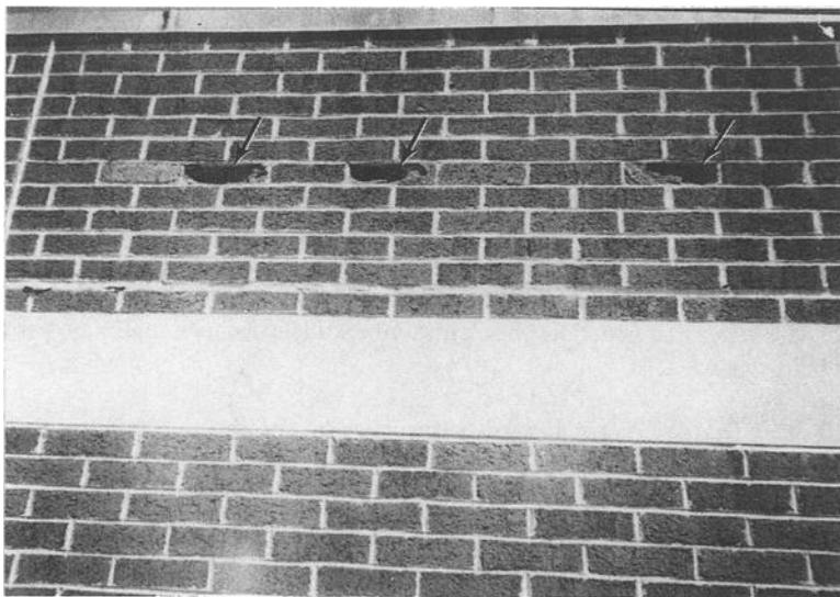
Figure 1--View of spalled dubrick due to cyclic freezing of saturated brick
