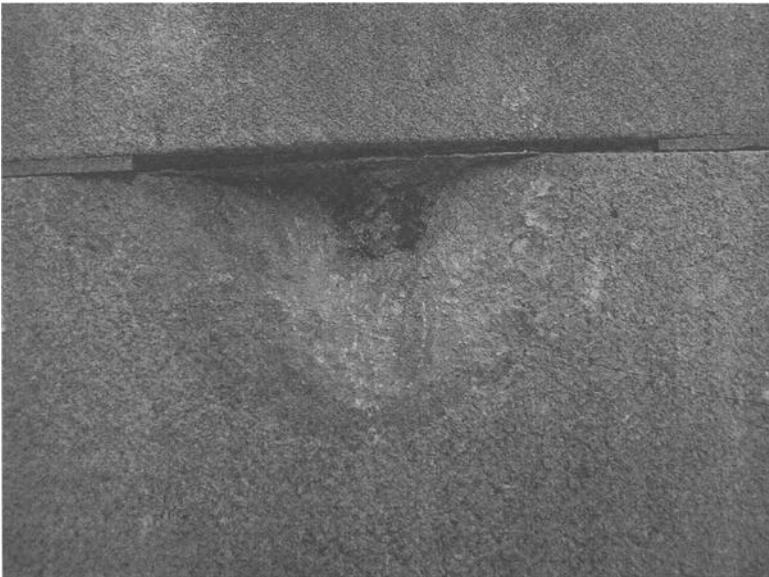
Figure 6 – Localized spalling caused by corrosion of embedded anchor
