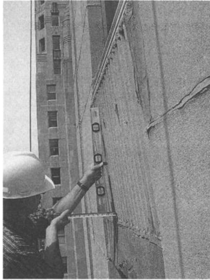
Figure 11 – Checking plumbness of limestone panel
