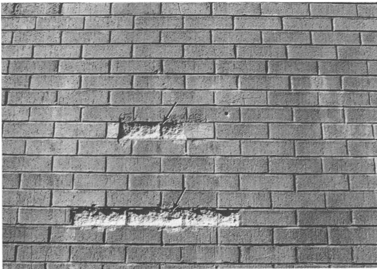
Figure 6--View of spalled brick due to cryptoflorescence behind coating on brick
