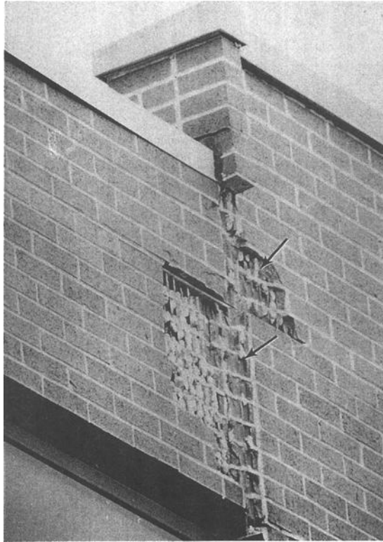
Figure 11-- View of spalled brick due to horizontal compressive stresses in wall
