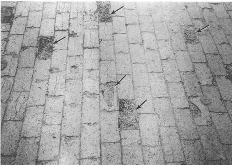
Figure 2--View of spalled paving brick due to cyclic freezing of saturated brick
