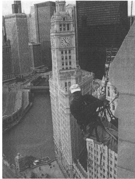
Figure 10 – Inspection being performed by rappelling techniques
