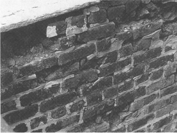
Figure 2 – Severe freeze-thaw damage of brickwork
