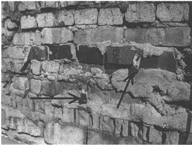
Figure 8 – Corroded lateral strap anchors
