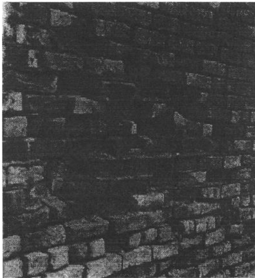
FIG. 2— Deteriorated wall on building constructed of Mexican handmade brick. [29]
