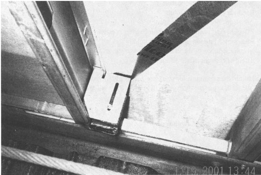
Figure 8 – Clip connection to floor angle.
