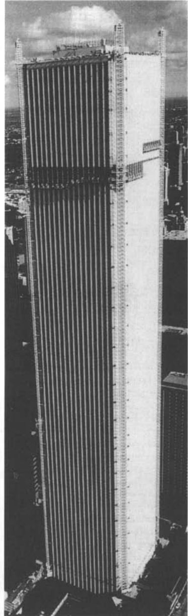
Chicago's Amoco Is Stripped of its Original Carrara Marble and Reclad in Granite. Only twelve years after its 1973 opening, periodic inspections found panels starting to bow outwards. By 1987, some of the 1¼ in. to 1½ in. thick 50 in. by 45 in. marble panels had bowed 1½ in.. More than 44,000 panels were replaced while occupants worked inside.
