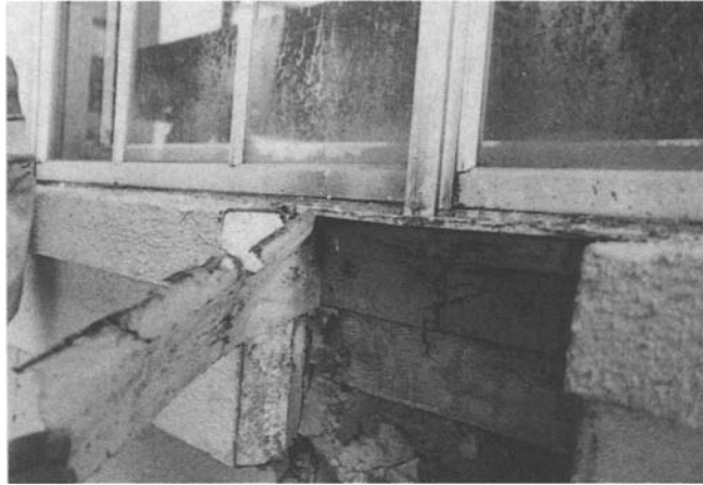
Figure 11 – Remnant of Polyethylene Installed Over Windows Prior to Stucco Application
