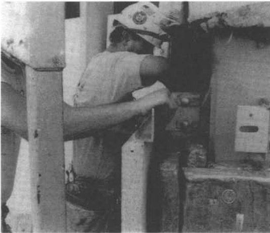
Chicago's Amoco Is Stripped of its Original Carrara Marble and Reclad in Granite. Only twelve years after its 1973 opening, periodic inspections found panels starting to bow outwards. By 1987, some of the 1¼ in. to 1½ in. thick 50 in. by 45 in. marble panels had bowed 1½ in.. More than 44,000 panels were replaced while occupants worked inside.
