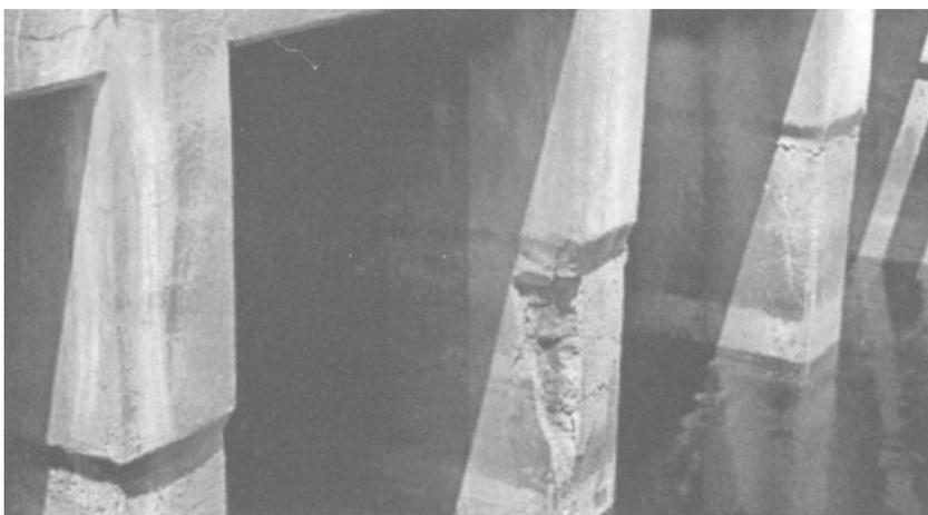
Figure 12-*Spalling of concrete due to corrosion of steel reinforcement in the unprotected areas of seawater structure #2.*
