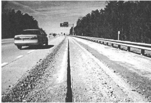
Figure 3- Overview of Trench and Drain Panel.
