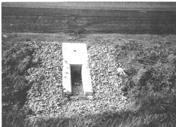
Figure 3 - No. 2 placed around the headwall.
