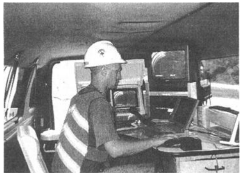
Figure 6 - Contractor personnel recording and logging edge drain (QC) inspection from inside of inspection vehicle.
