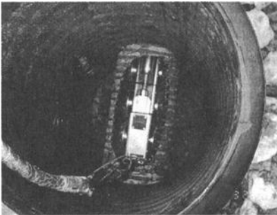
Figure 10 - Pipeline camera inspecting 8-inch collector pipe.
