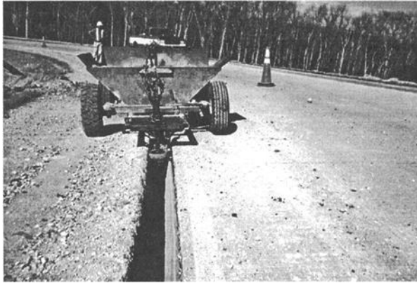
Figure 5- Drain Panel Positioning Wheel.
