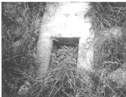
Figure 2 - Clogged headwall.
