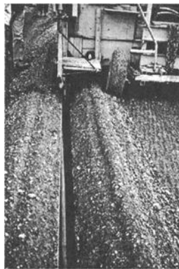
Figure 4- Drain Panel Positioning Plate.
