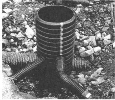
Figure 9 - Construction of ditchline collector system, and vertical inspection port.
