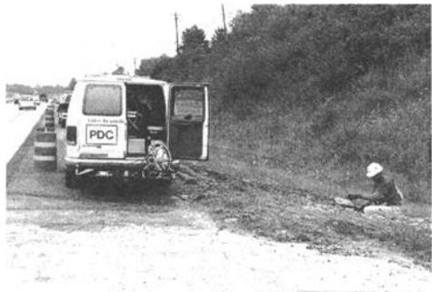
Figure 5 - Contractor personnel pushing camera into edge drain outlet for QC inspection.
