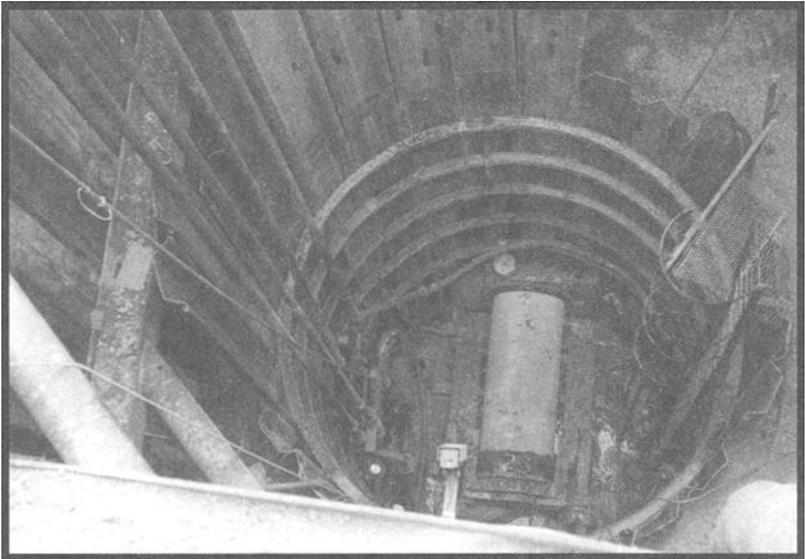
*Figure 8 -- Pipe positioned in jacking cradle at second shaft.*
