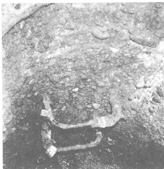
FIG. 3—Corroded manhole of ordinary Portland concrete, Arcachon sewer, France.
