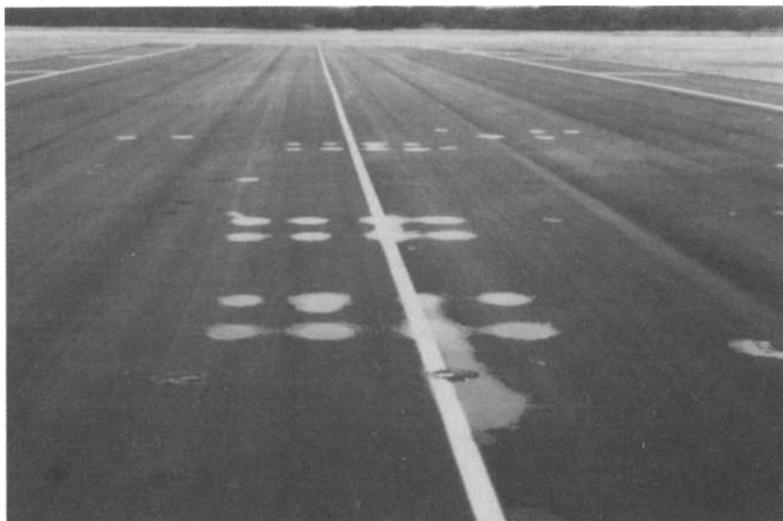
FIG 1.--Depressions resulting from parked aircraft.
