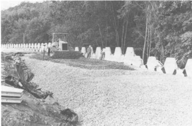
FIG. 2--Photographs of wall construction and geosynthetic layout.
