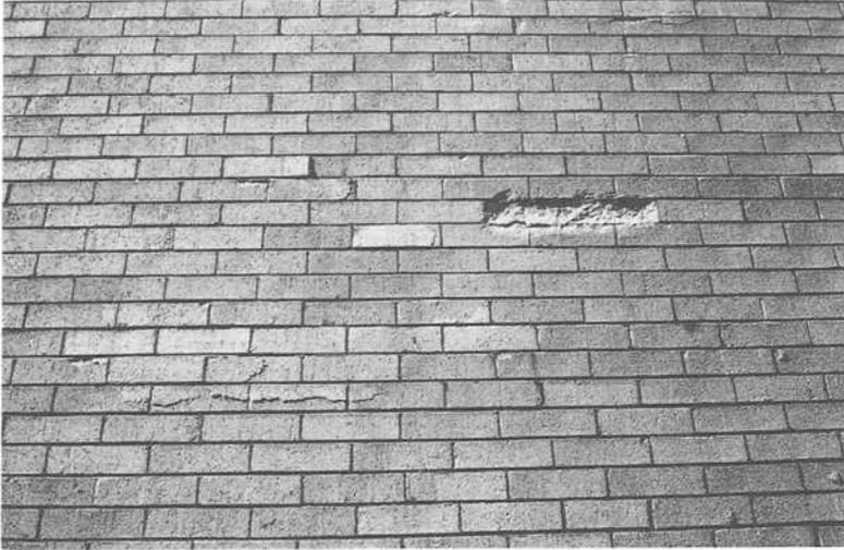
Fig. 3 - Spalling of bricks due to efflorescence build-up behind "water repellent" coating
