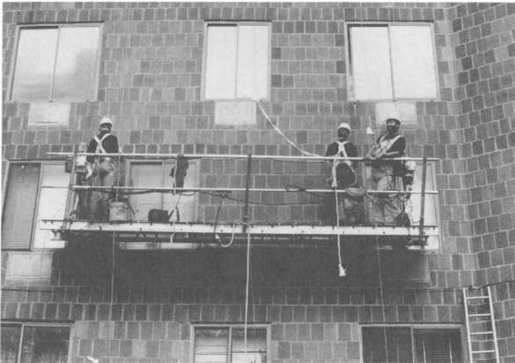
FIG. 4--Photograph of Inspectors at a Scaffold Drop Location
