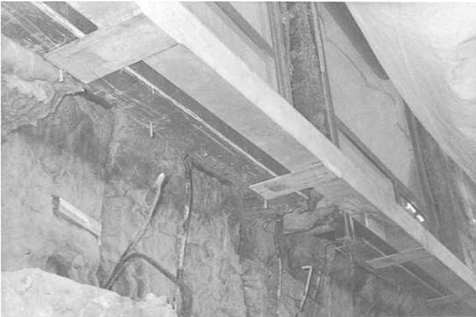
FIG. 4--Tabs on temporary aluminum support tube extend beneath window sill frame.
