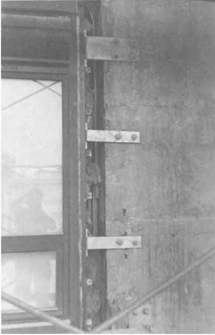
FIG. 2--New attachment clips between concrete column and window jamb.
