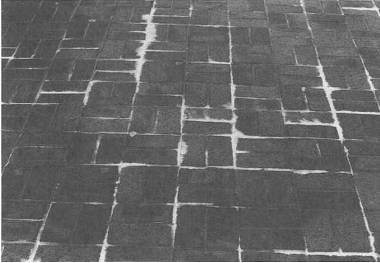
Fig. 6 - View of efflorescence on brickwork pavement
