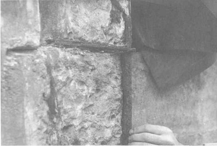
FIG. 6--Deterioration of concrete frame and corrosion of reinforcing steel.
