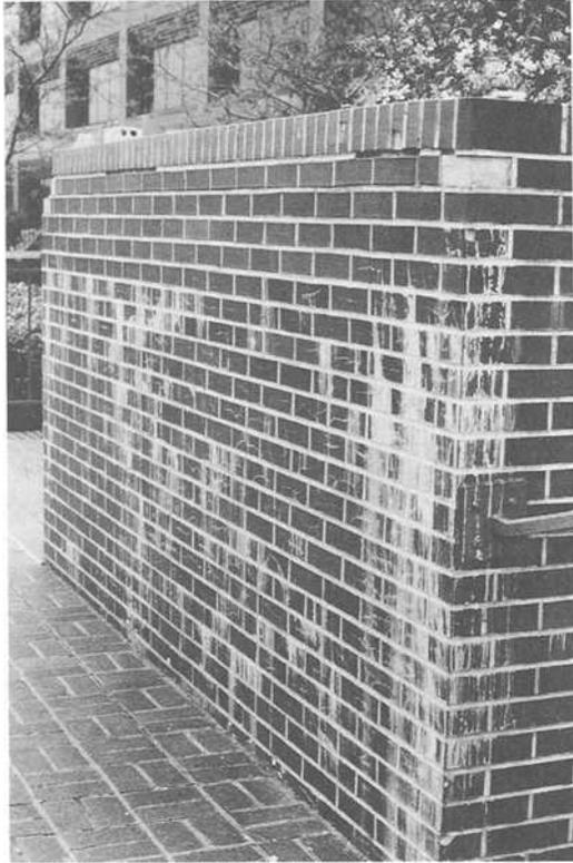
Fig. 5 - View of efflorescence below brickwork coping
