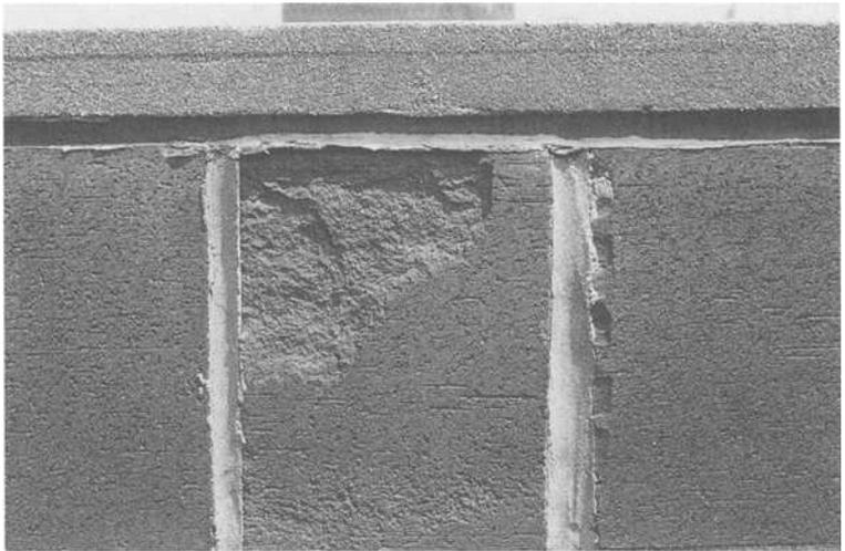
**FIG. 3--Spalled Tile at Parapet Coping**
