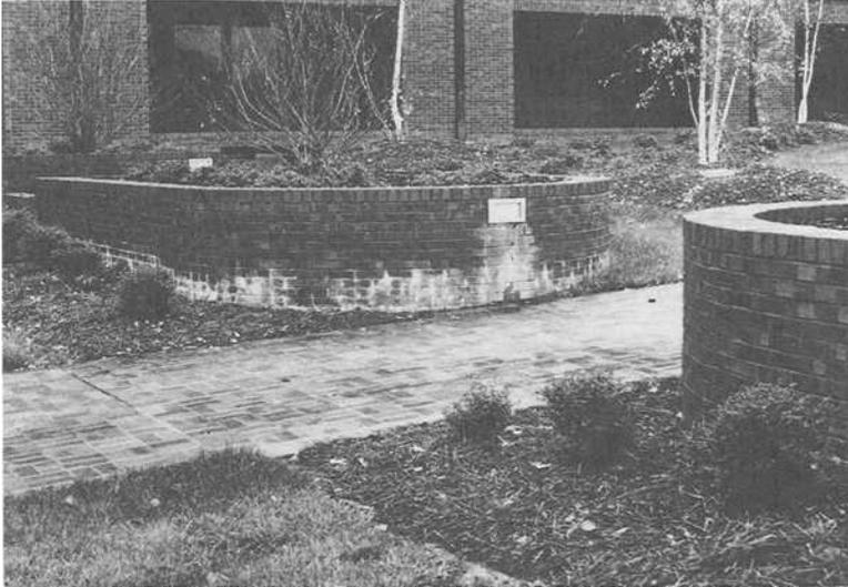
Fig. 7 - View of efflorescence on brickwork planter box
