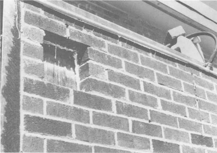
Fig. 5 -- Water spray at top of test panel
