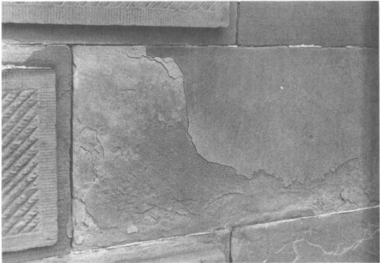
Fig. 5 -- Typical delamination of sandstone units.
