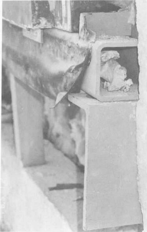
FIG. 5--Permanent steel tube in place beneath window sill with uncured neoprene membrane flashing.
