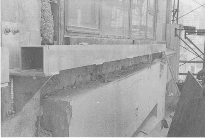
FIG. 3--Temporary aluminum support tube mounted in front of window sill.
