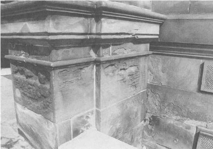
Fig. 7 -- Severe deterioration of sandstone at south entrance.
