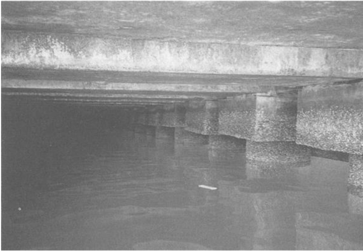
Figure 5. General Condition under wharves (Note barnacle line on pile caps).
