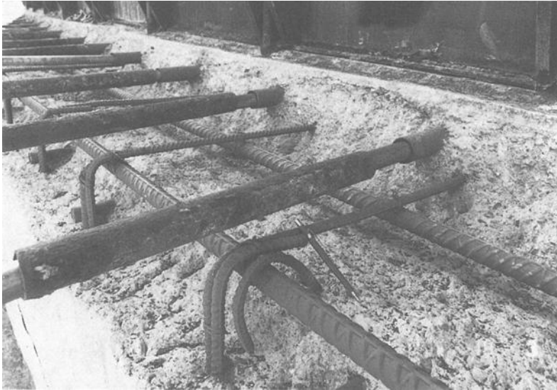
FIG. 2--Preparation of embedded steel and concrete for repairs.
