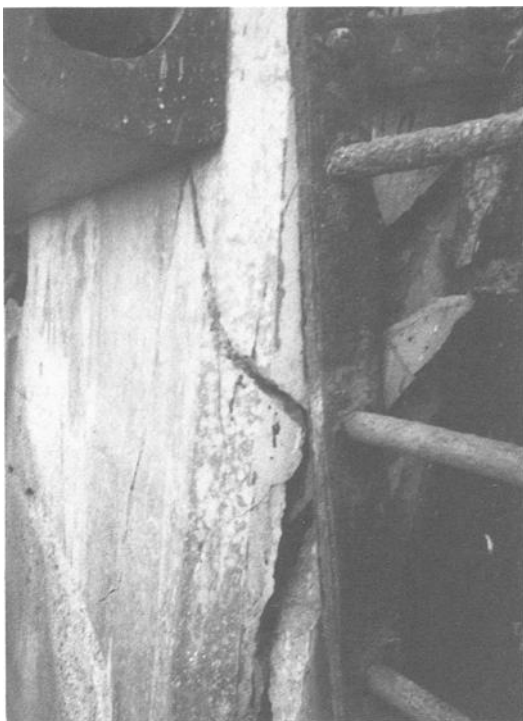
Figure 6. Cracks formed at Ladder recess.
