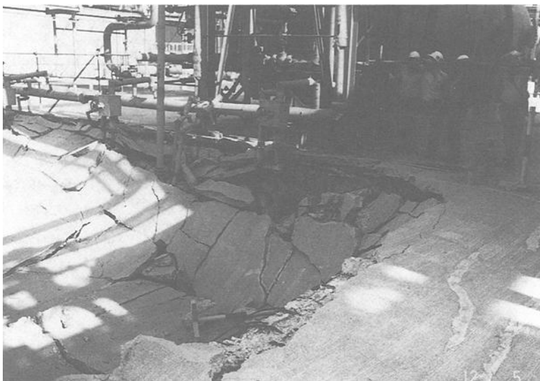
FIG. 6--Collapse of the sulfur pit roof slab.
