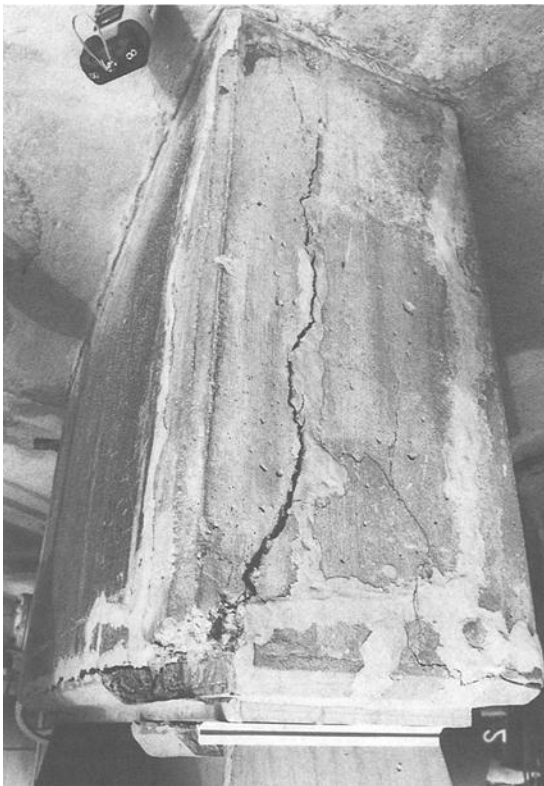
FIG. 7--Deteriorations in a typical vessel support.
