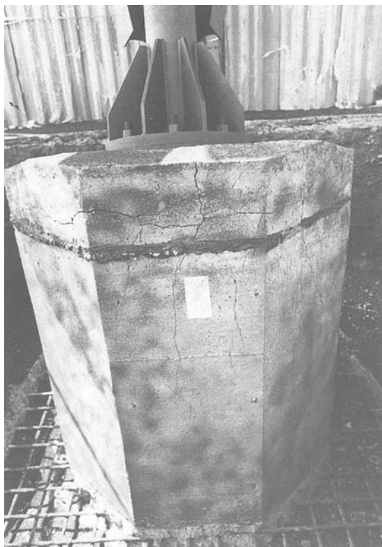
FIG. 3--Cracking of concrete cover in the plinth.
