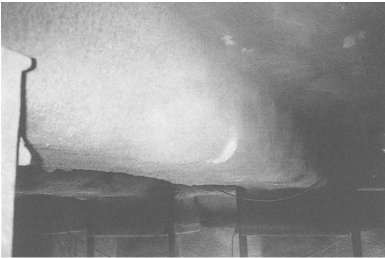
Figure 11. Condition of beam after repair and installation of anode in sprayed concrete overlay.
