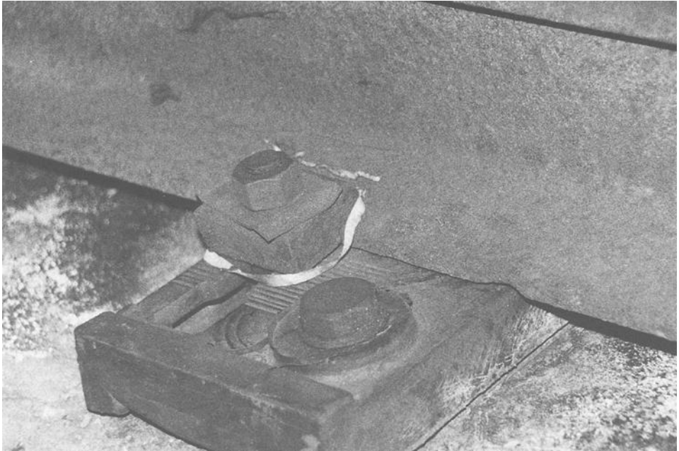
Figure 4. Photograph of Fastener on BART System with Notch in Rail due to Corrosion.
