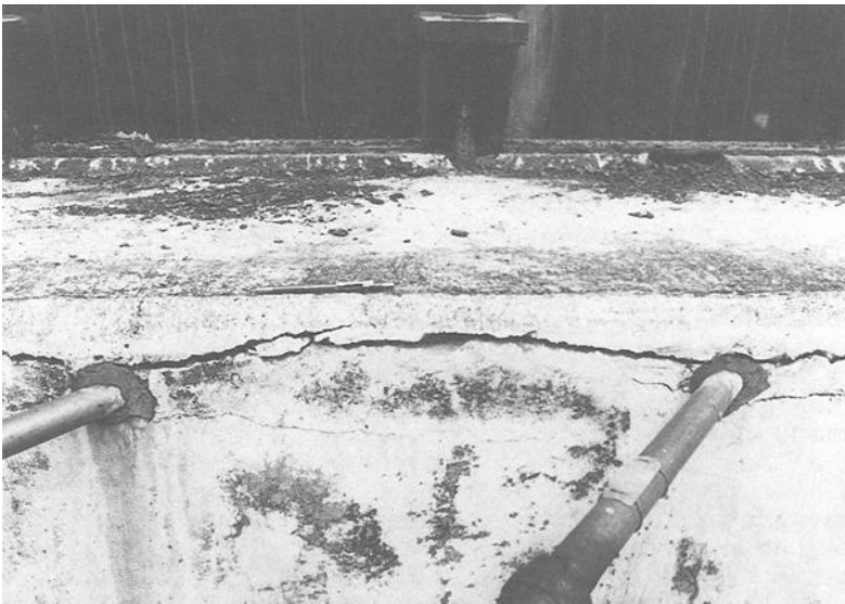
FIG. 1--Deterioration of concrete in areas of the heater tubes.
