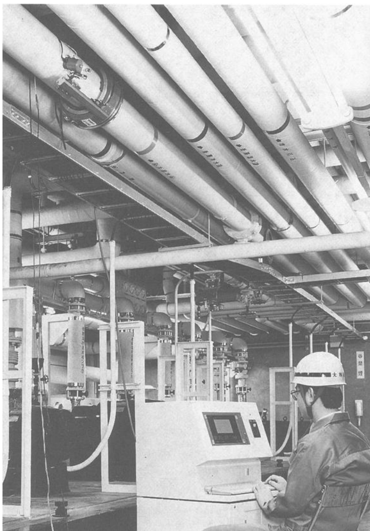
PHOTO. 1 -- Field measurement using pipe inspection robot.
