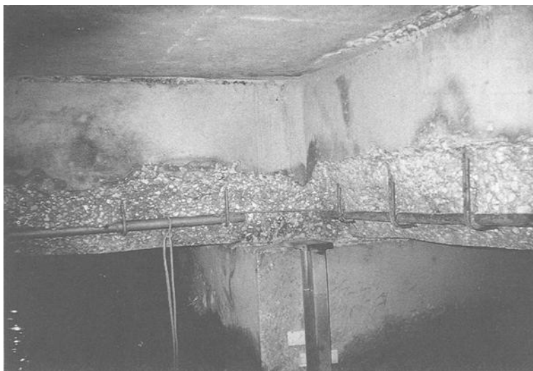
Figure 9. Damaged lower corner of beam removed and blast cleaned. Bonding straps installed between beams
