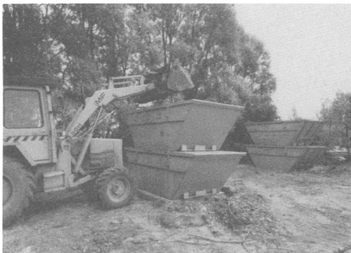
Fig. 5b Sand filled skips in place
