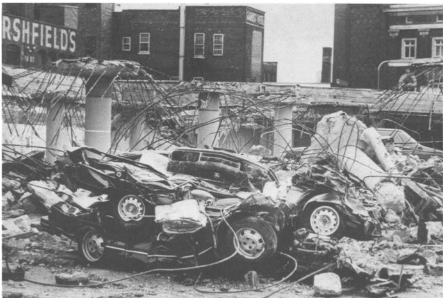
FIG. 2— Collapse of a salt-damaged parking garage [6].
