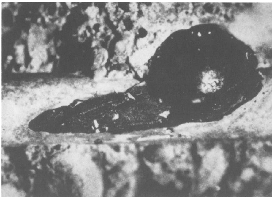
FIG. 7—Corrosion at void in concrete [60].
