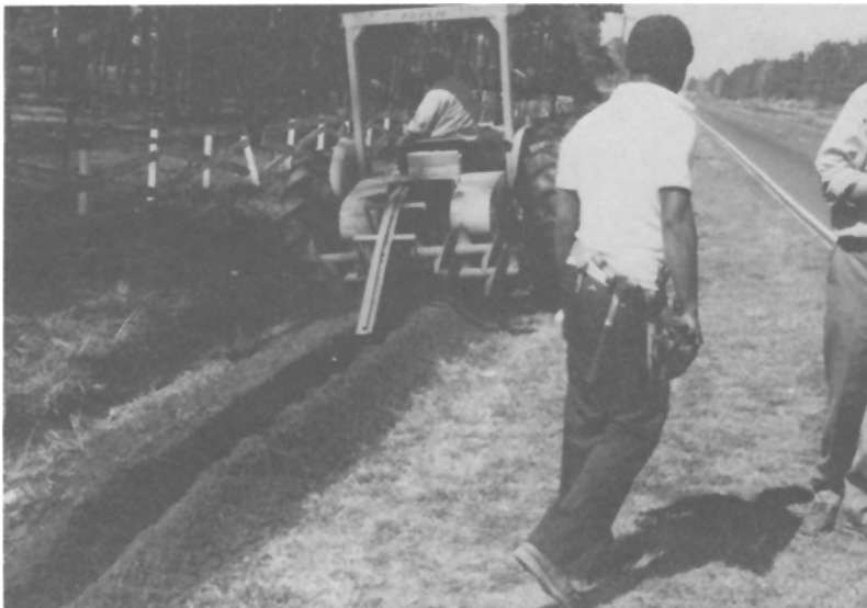
FIG. 4—Telephone cable is trenched in for field service corrosion tests on metallic shields.
