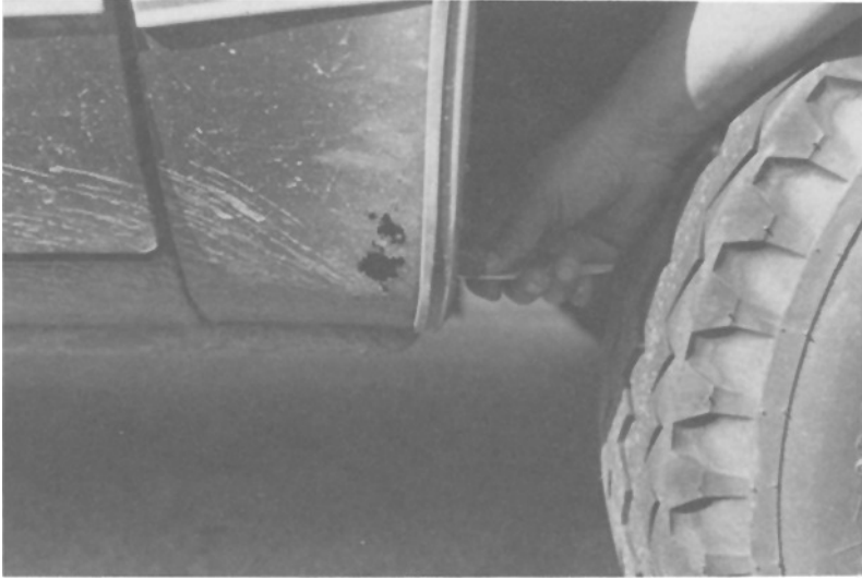
FIG. 3—Perforation corrosion of auto-body panel is caused by accumulation of poulitice, which traps salt and acids.
