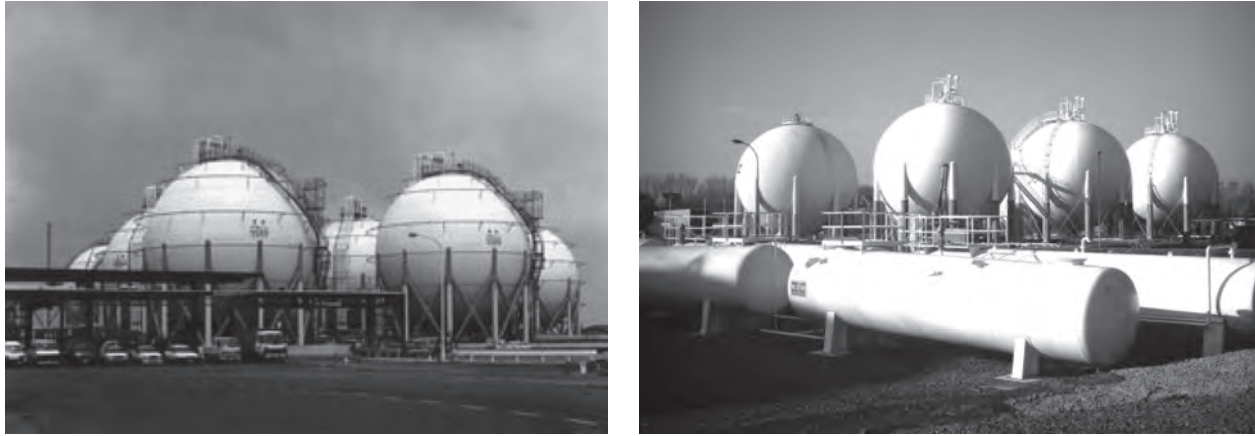
Figure 20.5—Spherical and horizontal bullet tanks. Source: [1].
