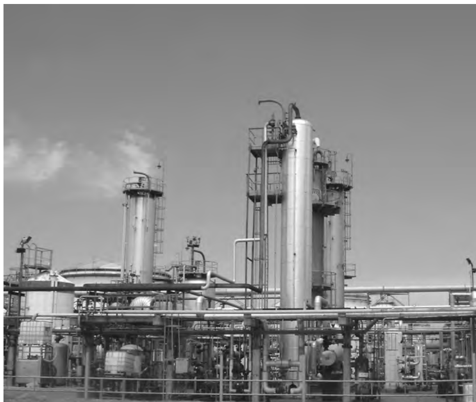
Figure 11.3 —Amine unit at the YPF La Plata Refinery (Argentina). Source: Picture courtesy of YPF.
