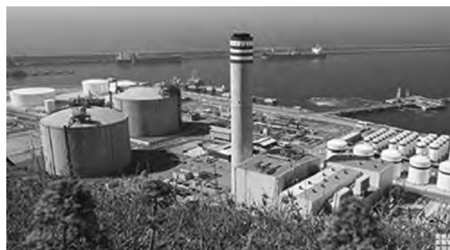
Figure 11.21 —LNG import terminal integrated with a power generation plant (BBG-BBE). Source: Picture courtesy of Bahía de Bizcaia Gas, S.L.
