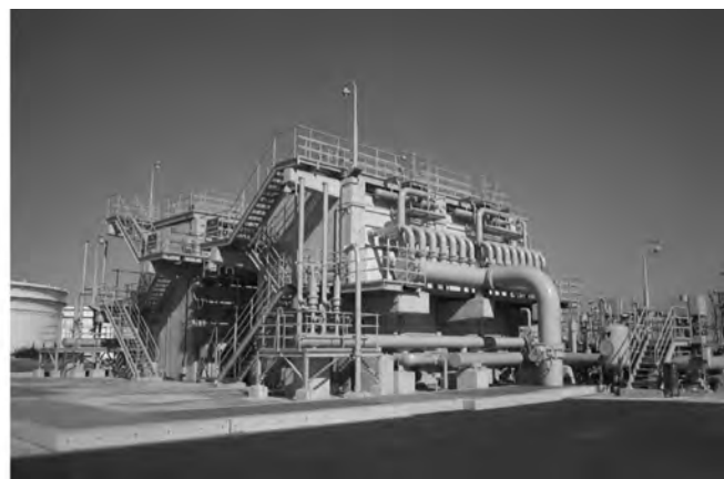
Figure 11.19—ORV at Sumitomo Precision Products, Co., Ltd. (left) and Tokyo Gas, Co., Ltd. (right).
