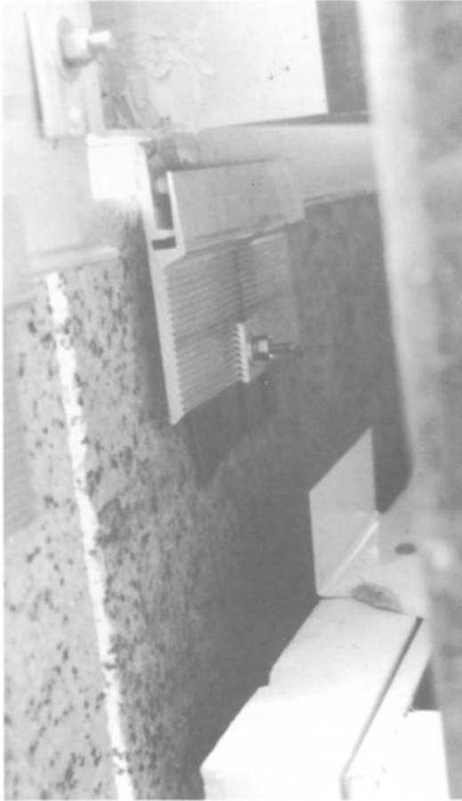
◀ FIGURE 50: *Movement Accommodation Between Floors.* Horizontal movement joints accommodate differential long and short-term movements between floors. As the skin moves, the stone anchorage must accept the dynamics without transferring movement or force into the stone panel. Here, a flange extends down from the extruded window sill that engages a grooved clip. The serrated leg allows for adjustments and tolerances to provide the proper safe engagement.
