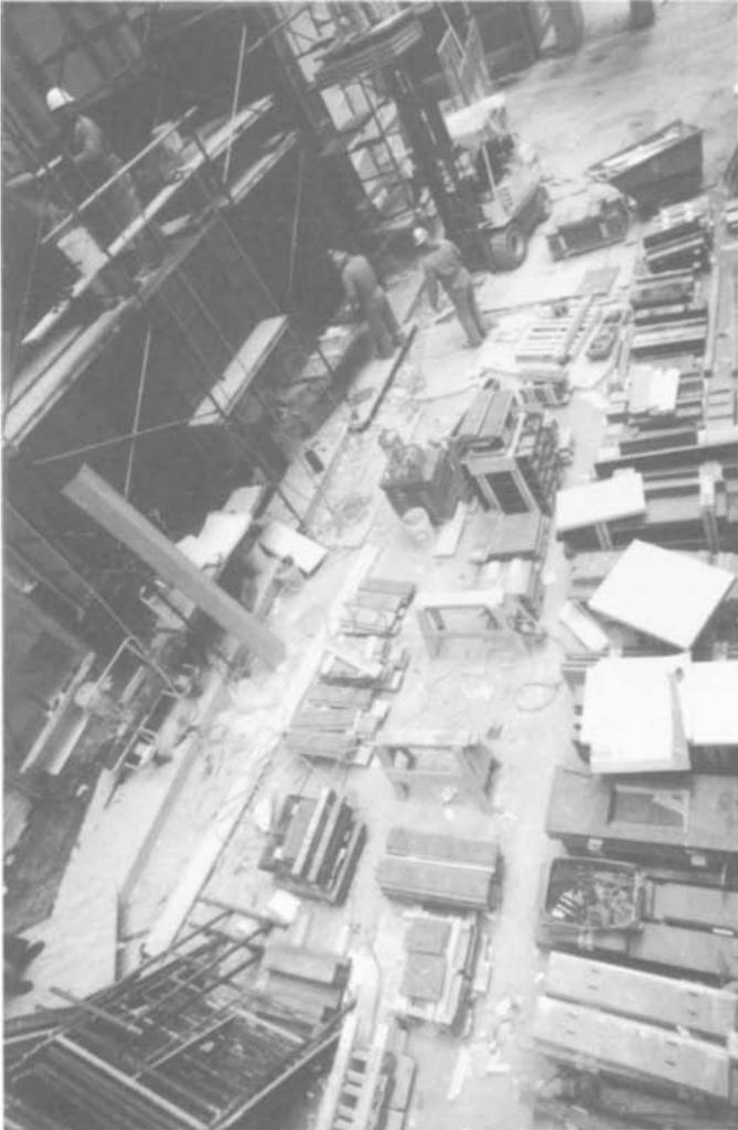
▲ **FIGURE 60: *Ground Floor Entrance Stone Shake-Out.*** At the entrances, where few of the stone panels were typical or repetitive, significant area was required to uncrate and shake-out materials. Since the entire width of the entrance was scaffolded, several crews worked simultaneously to erect the base. Multiple crews in different areas also required more crates to be open and available at the same time. Stones are usually crated by similar sizes and types in nontypical areas.
