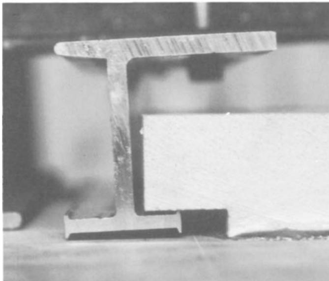
FIGURE 93: *Kerfed Liner Block Anchor*. Side view of the anchor engaging the block attached to the back of the face stone in a soffit condition.
