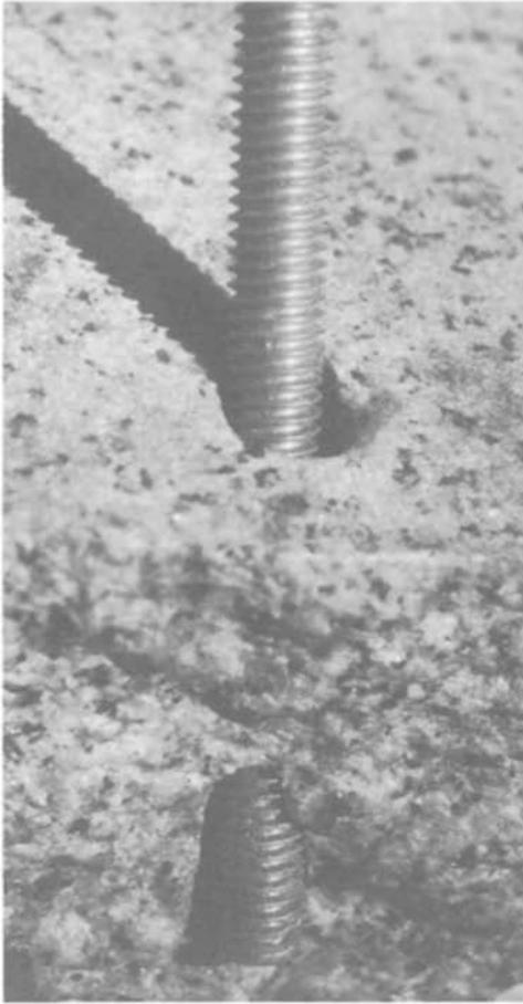
◀ FIGURE 73: *Inclined Dowel Anchor In Stone.* Where stone panels are supported on precast panels or will be secured to trusses with grout pockets, a threaded rod engages an inclined hole drilled into the back of the stone. Take care to attain sufficient engagement, yet maintain sufficient cover on the exposed face. Bed the rod in compressible fill, sheath the back of the stone with a bond-breaking slip-sheet, and use of rubber grommet on the threaded shank for proper anchor performance.
