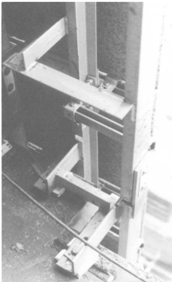
support when the top edge of the stone is inaccessible.
