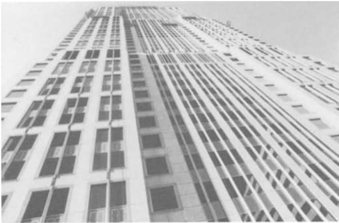
◀ FIGURE 55: *A T & T Chicago’s Facade Under Construction.* In comparison to the mock-up shown in Figure 23, the typical areas of stone remain unchanged in stone type, finish, and joint configuration. Three swingstages near the top of the second set-back at the 47th floor continued the steady ascent to the roof. Above that, the aluminum curtainwall framing preceded before the stone, due to the stone being mullion-supported.
