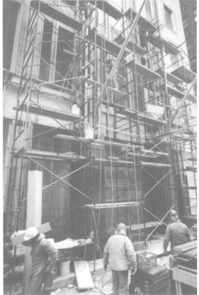
▲ **FIGURE 61: *Ground Floor Entrance Stone Installation.*** With the three-floor-height entrance scaffolded, workmen on the top levels finalized the alignment of the prefabricated aluminum framing system while setters placed stone onto that framing near the top of the first floor. This is the entrance to the “bussel” connector between A T & T and what is now U S G.
