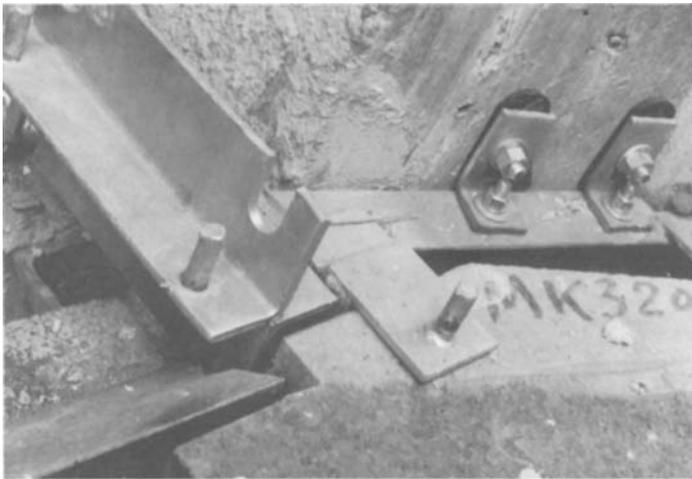
▲ **FIGURE 69: Pin Anchorage at Entrance Arch Stone Moulding.** A pinned bracket attaches to the contoured stone moulding to provide positive mechanical engagement. This bracket allows for attachment of equipment during erection as well as final adjustment of the stone relative to the concrete building frame backup.
