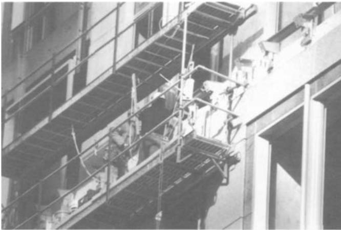
▲ FIGURE 58: *Exterior Swingstage For Cladding Installation.* Work platforms were suspended from monorails cantilevered through the openings above. These platforms held the men, tools, and miscellaneous parts needed to install the stone cladding. A solid platform above provided overhead protection from curtainwall and structural building frame construction that continued above.
