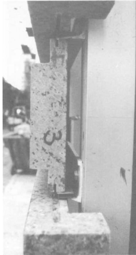
▲ FIGURE 66: *End View of Kerf Anchor In Stone Panel.* Using the same system shown in Figure 65, this view shows the stone engaged by the clip at the kerf, and the clip attached to the pre-aligning backup frame. Note the plastic setting shim used for leveling the stone and the bolted connection between the clip and the backup
