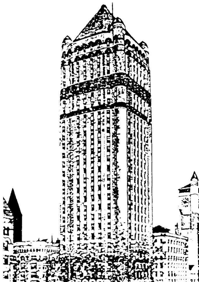
▲ FIGURE 8: *“Cloudscraper” Proposal (1887)*. Applying the patented iron framing system, Leroy Buffington proposed construction of a 28-story tower. Made possible in concept by using the iron construction techniques learned from Gustav Eiffel, this idea revolutionized the approach to structure for American high-rise buildings. Drawing from *Inland Architect and News Record* 11 July 1888.
