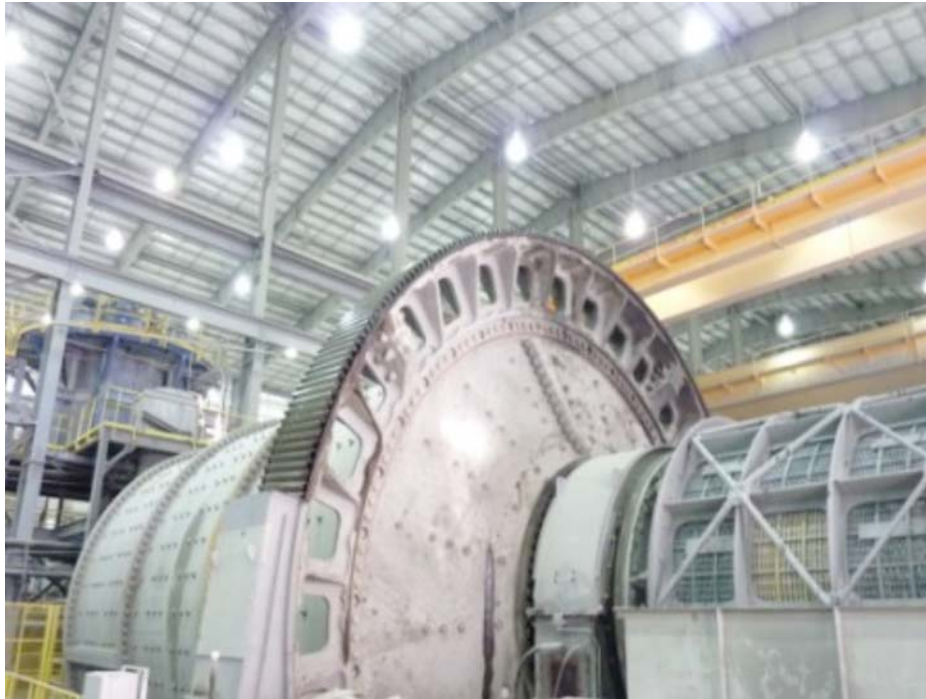
FIG. A1.1 Cleaned Girth Gear Ready for Examination
