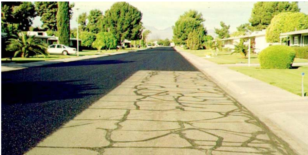
FIG. X1.1 Example of Block Cracking Due to Aging
