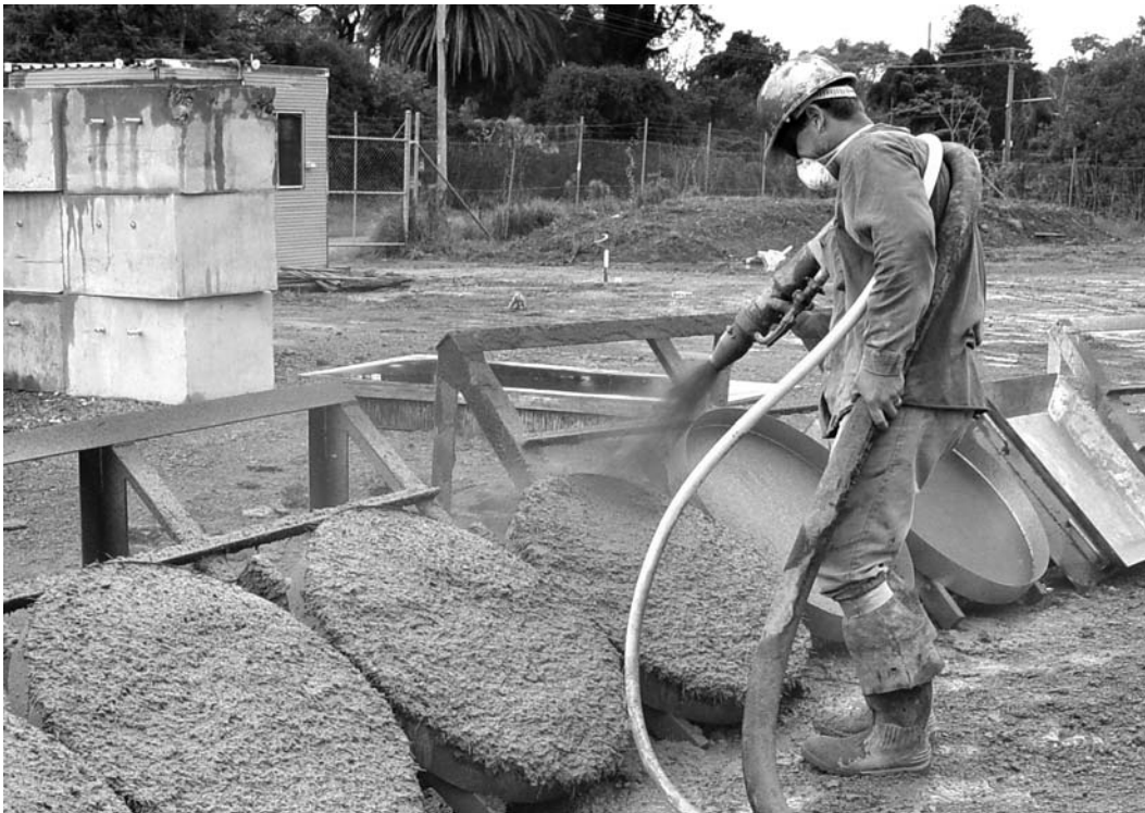
FIG. X1.5 Manual Spraying of Panels
