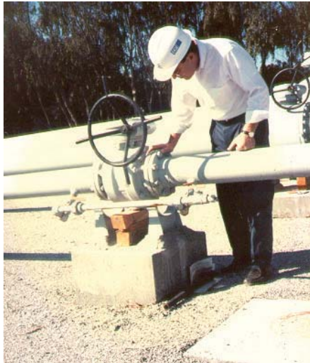
Figure 25 - Ground Liquefaction Causes the Saddle Supports to Sag Down, Pipe Did Not Fail
